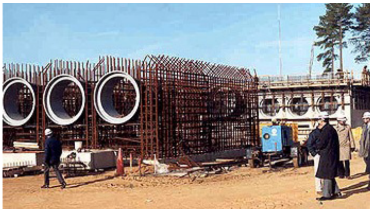
NUHOMS horizontal spent fuel storage system under construction at the Calvert Cliffs Nuclear Power Plant in Lusby, MD.
