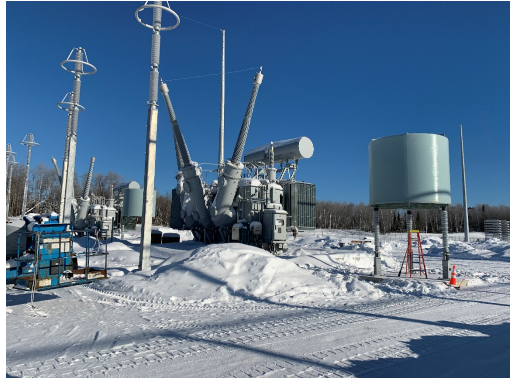
Neutral Ground Reactors Install
