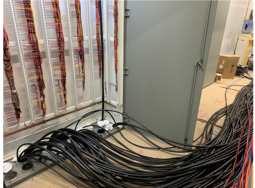
Cable pulls in EEE
