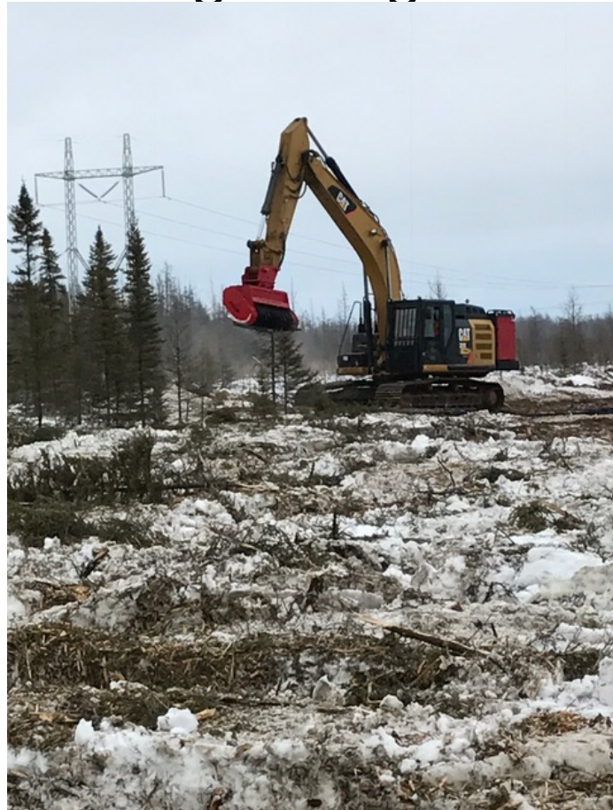
Clearing on Segment 2
