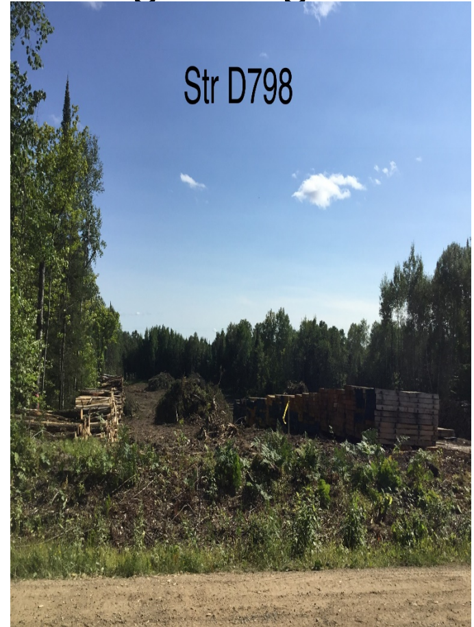
Clearing on Segment 4
