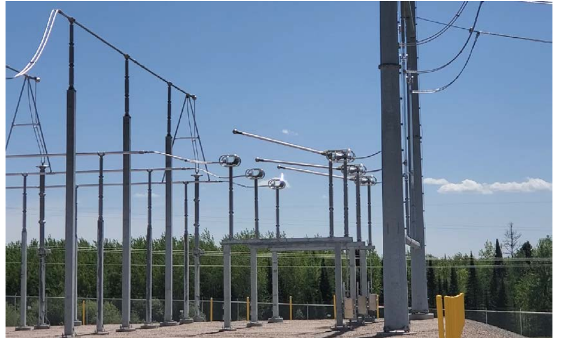
Electricity flowing on 3 rd switch
