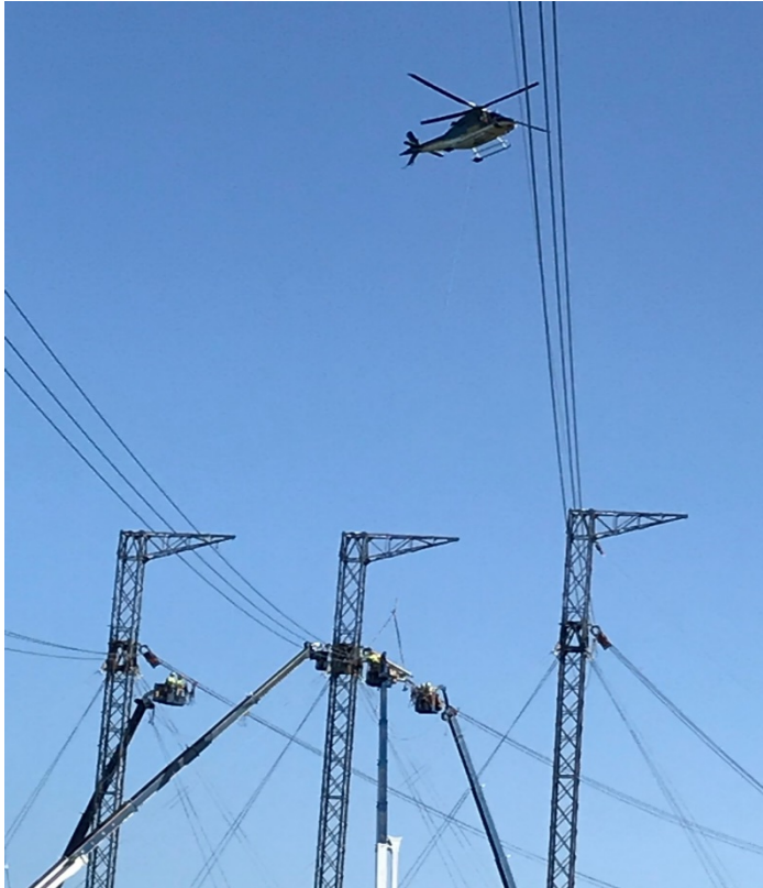
Stringing on Segment 4
