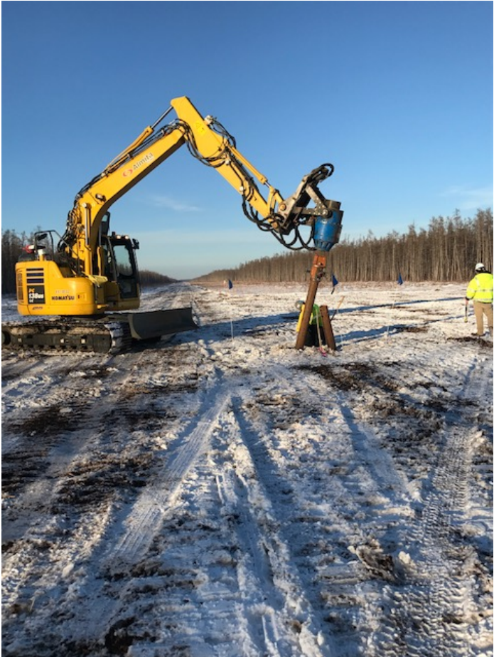
Helical Pile on Segment 1
