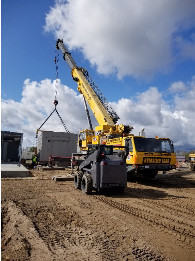
Install of EEE
