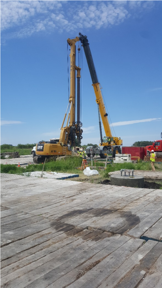
Drilled Piers on Segment 1
