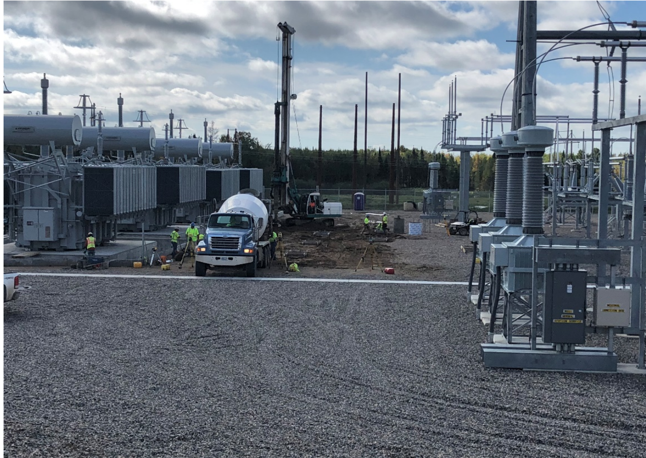
Drilled Piers in 230 kV Yard
