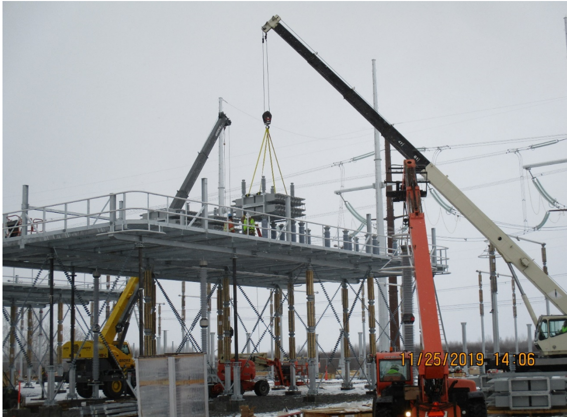
Capacitor Bank Install
