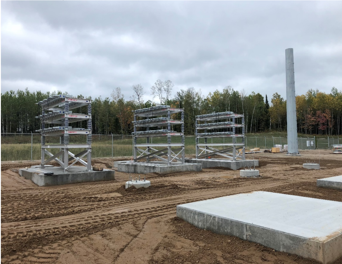
Cap Bank Erection
