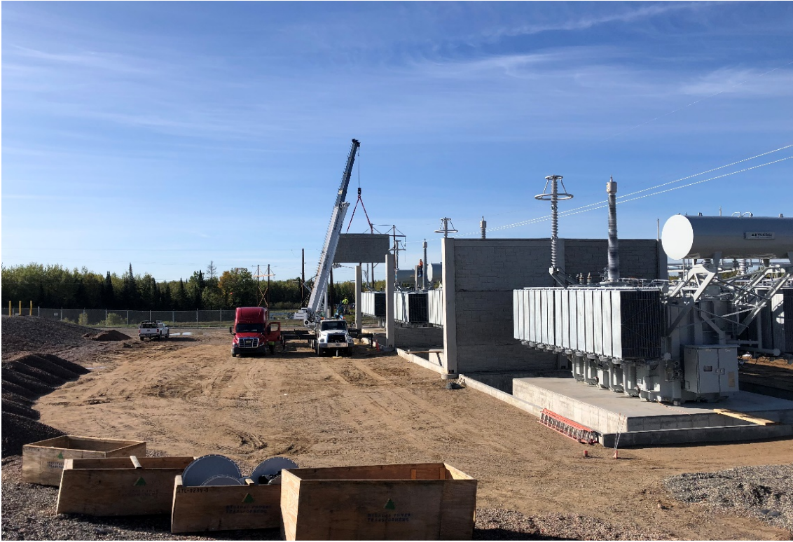
Transformer Firewall Installation
