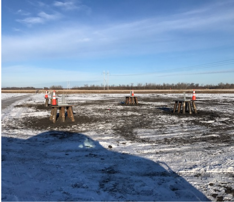
Complete Helical Pile Segment 1
