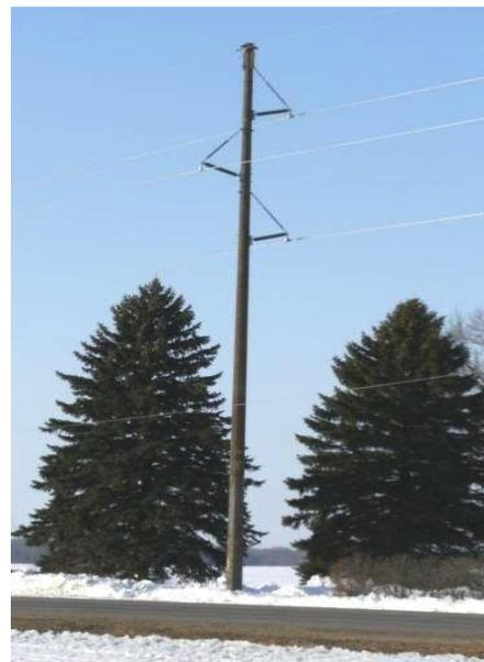
**Figure 7: Typical overhead gen-tie structure.**
