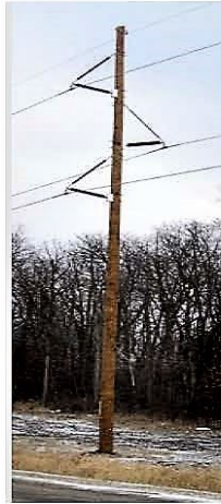
Diagram 3-2. Photos of Typical 115 kV Transmission Structures
