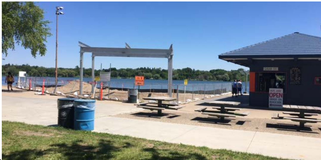
Photo 1: Installation of canopy structure to hold 7.380 kW DC array at Nokomis Park
