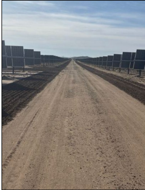
Figure 6: Typical ESS Access Road
