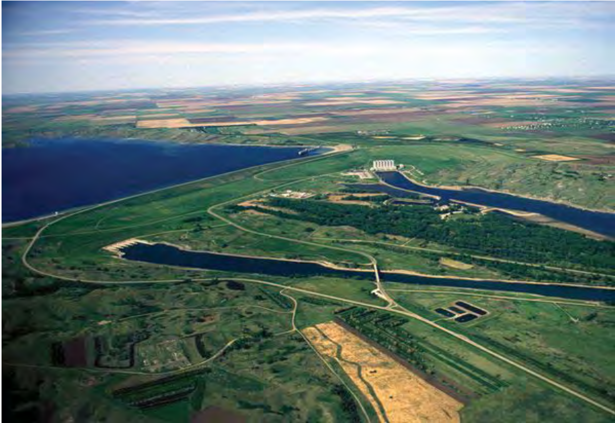
Aerial View of Oahe Dam on Lake Oahe near Pierre, SD 21
