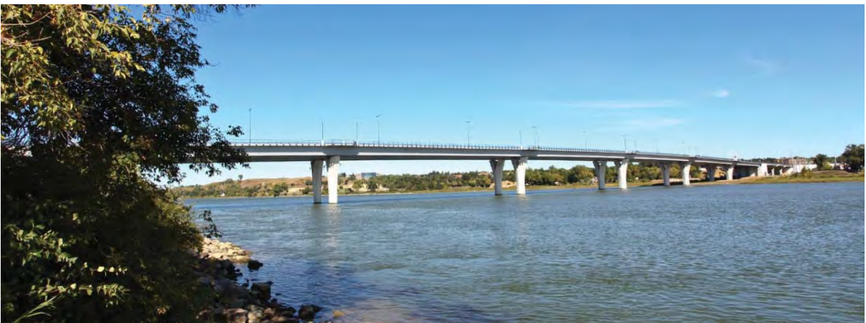
Coal ash was an additive in the concrete used to build the Memorial Bridge across the Missouri River in Bismarck, ND in 2008.
