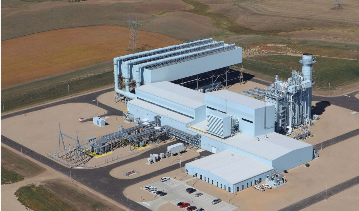
The Deer Creek Station near Brookings, SD, is Basin Electric's first natural gas-fired combined cycle power plant.
