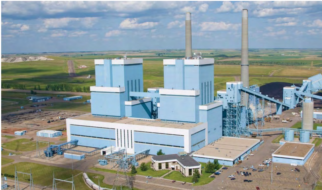
The Antelope Valley Station near Beulah, ND, is one of four coal-based power plants operated by Basin Electric. Its two units began commercial operation in 1984 and 1986.
