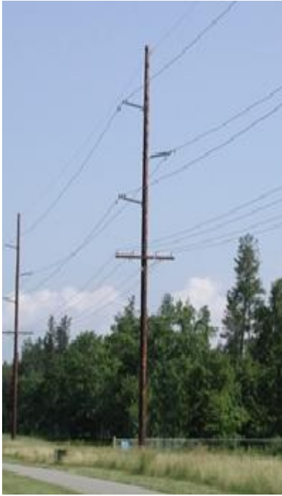
Typical Single Circuit with Underbuild
