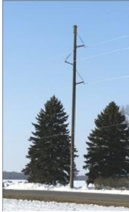
Typical Braced Post Structure
