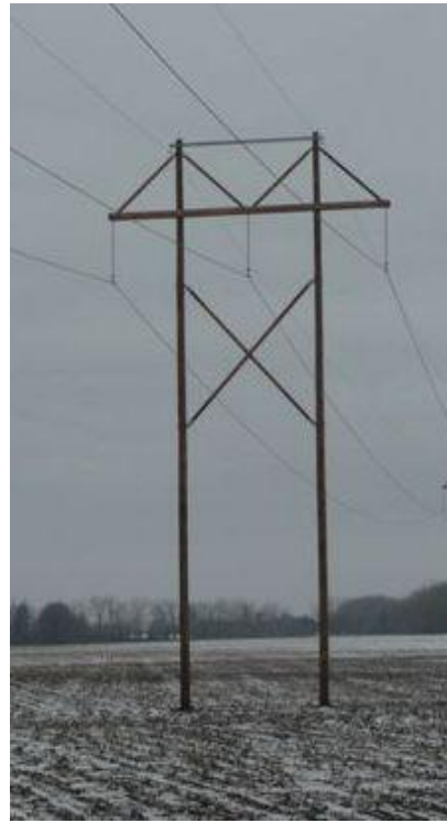
Typical H-Frame Structure
