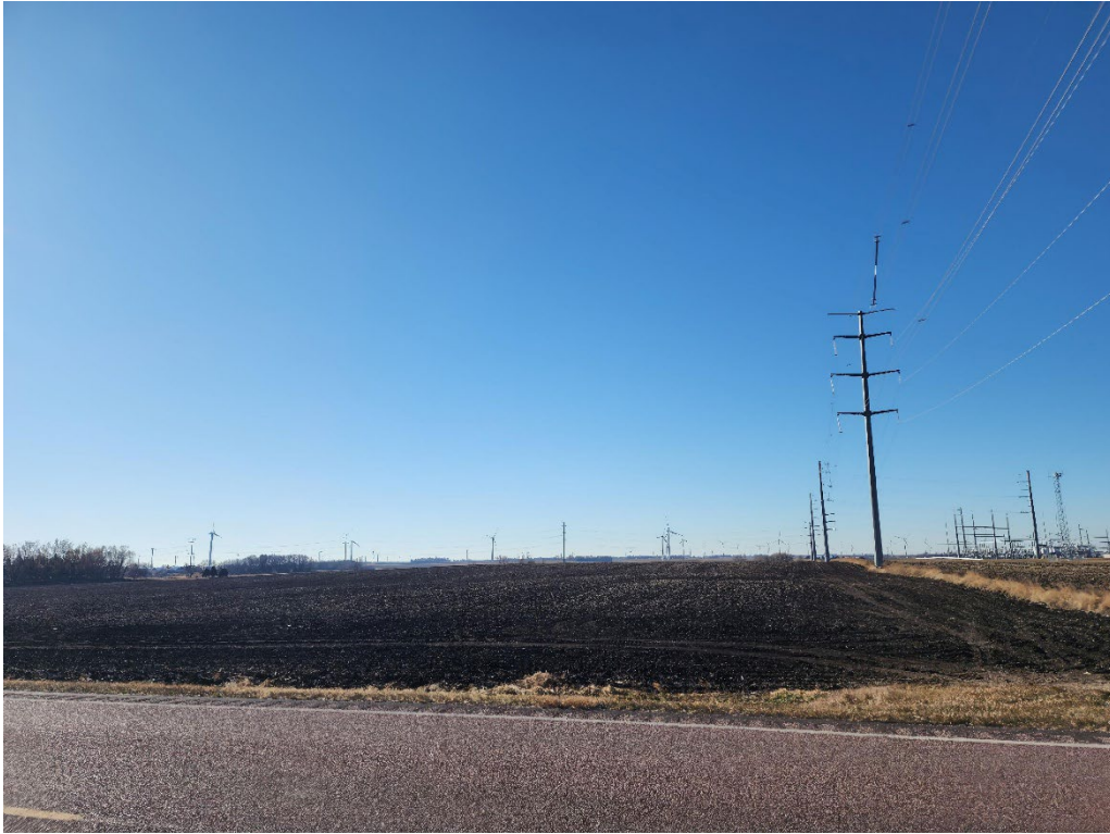
Existing view at McCall Avenue looking west.
