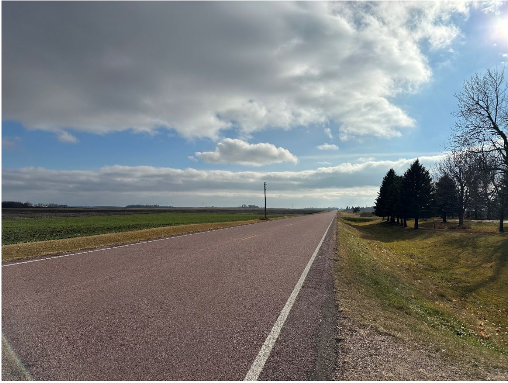
Existing view at McCall Avenue and 180 th Street looking south.
