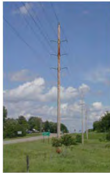
Typical Double Circuit 115 kV Structure
