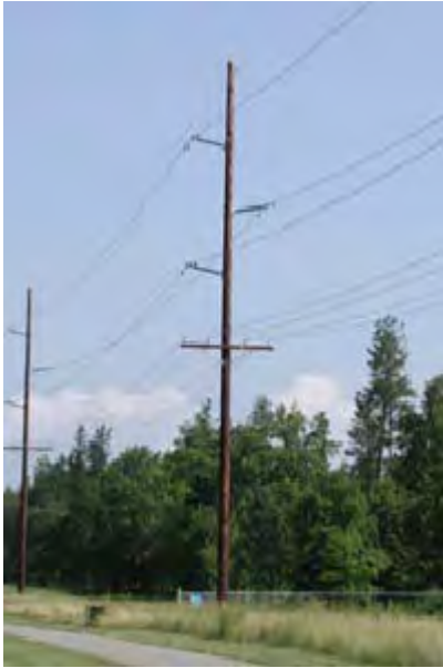
Typical Single Circuit Structure with Distribution Underbuild
