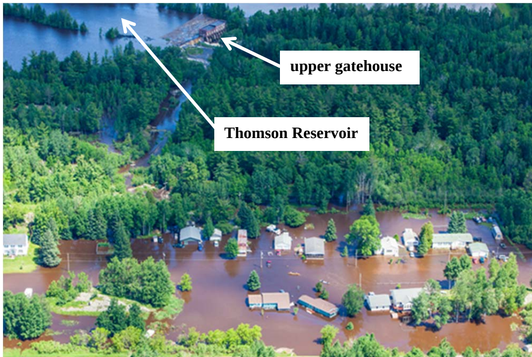
Figure 1. City of Thomson During the June 2012 Flood
