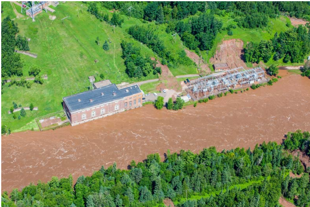
Figure 3. Thomson Powerhouse During the June 2012 Flood
