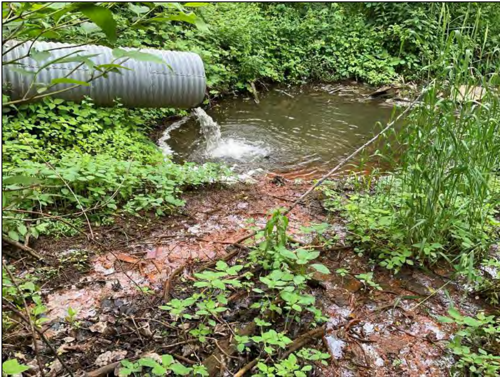
Photograph pp267 view North
