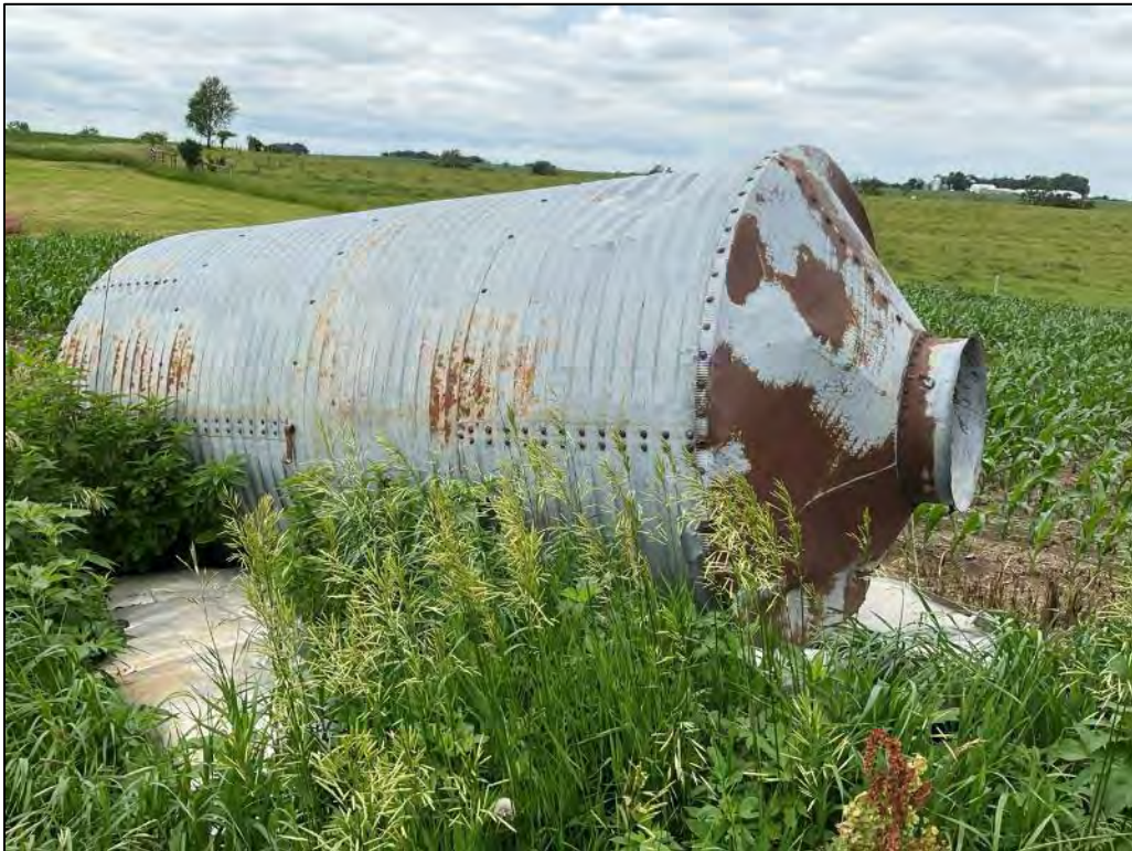
Photograph pp428 view of tank
