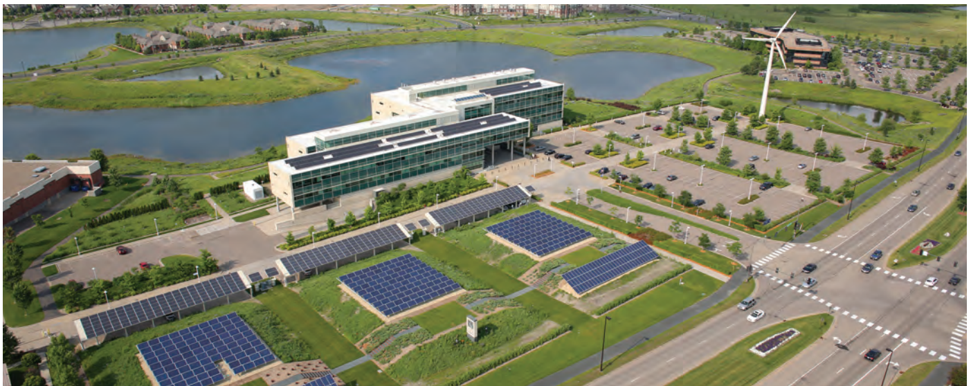
A variety of solar technologies and configurations are being tested at Great River Energy's headquarters site.
