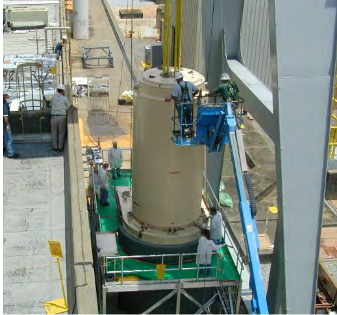
Figure C-16: Placement of Transfer Cask on Overpack with Mating Device
