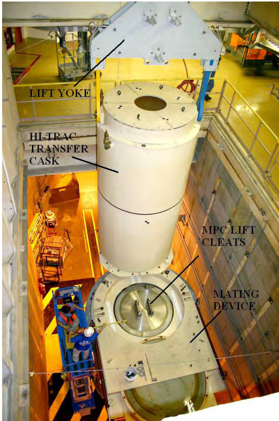
Figure C-15: Overpack, Mating Device, and Transfer Cask
