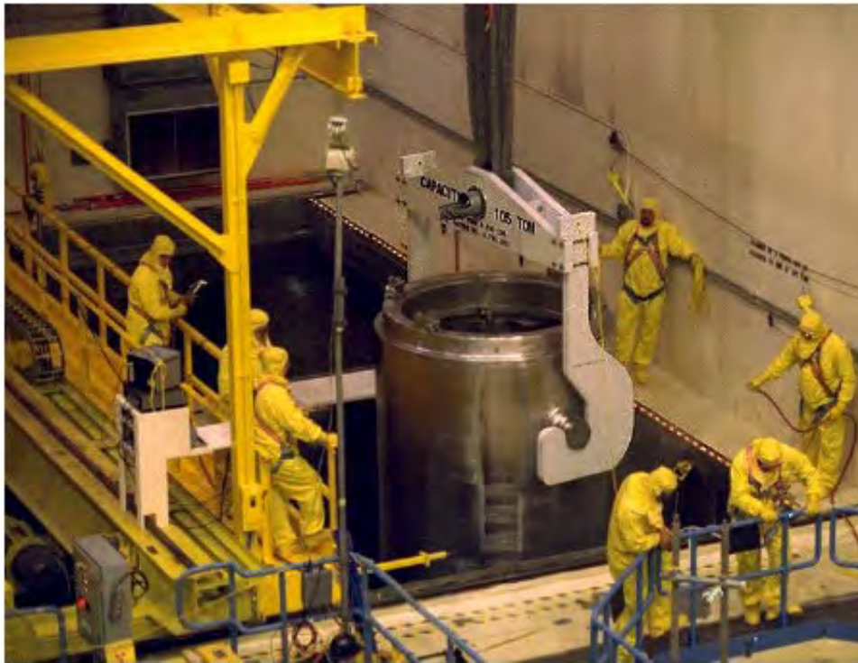
Figure 7. Canister and Temporary Metal Overpack Being Decontaminated
