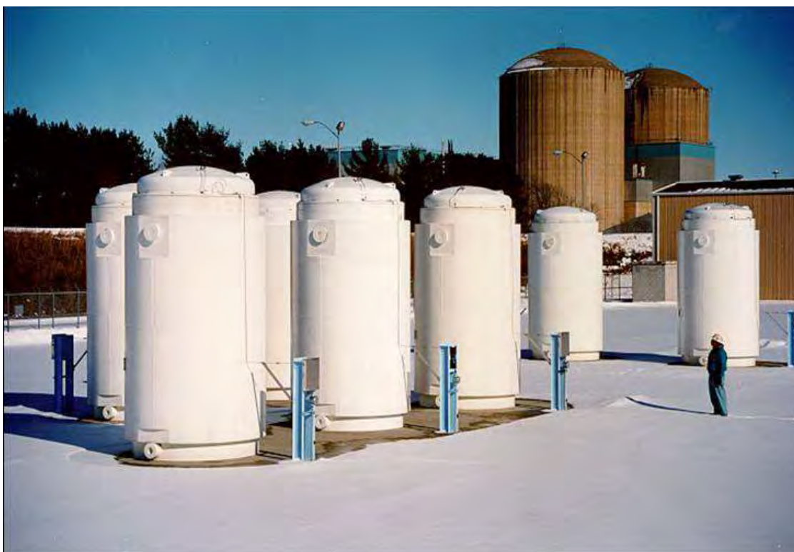
Figure 2. TN-40 Casks on ISFSI Pad
