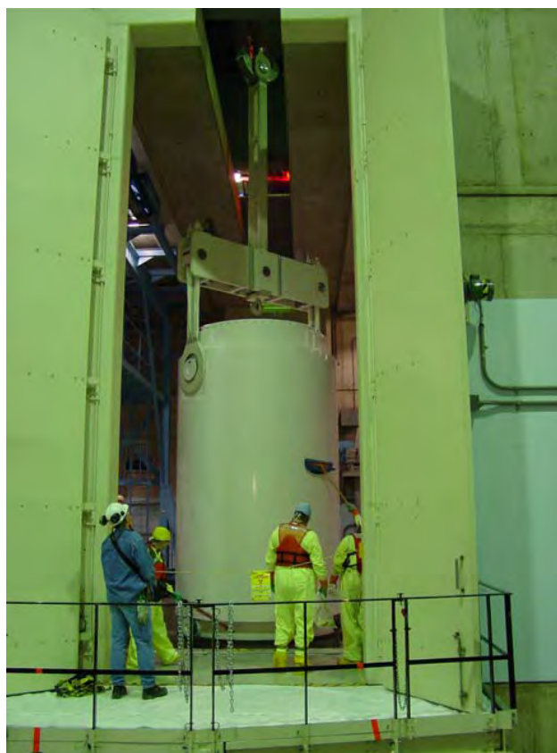
Figure 5. TN-40 Cask Removed from Spent Fuel Pool
