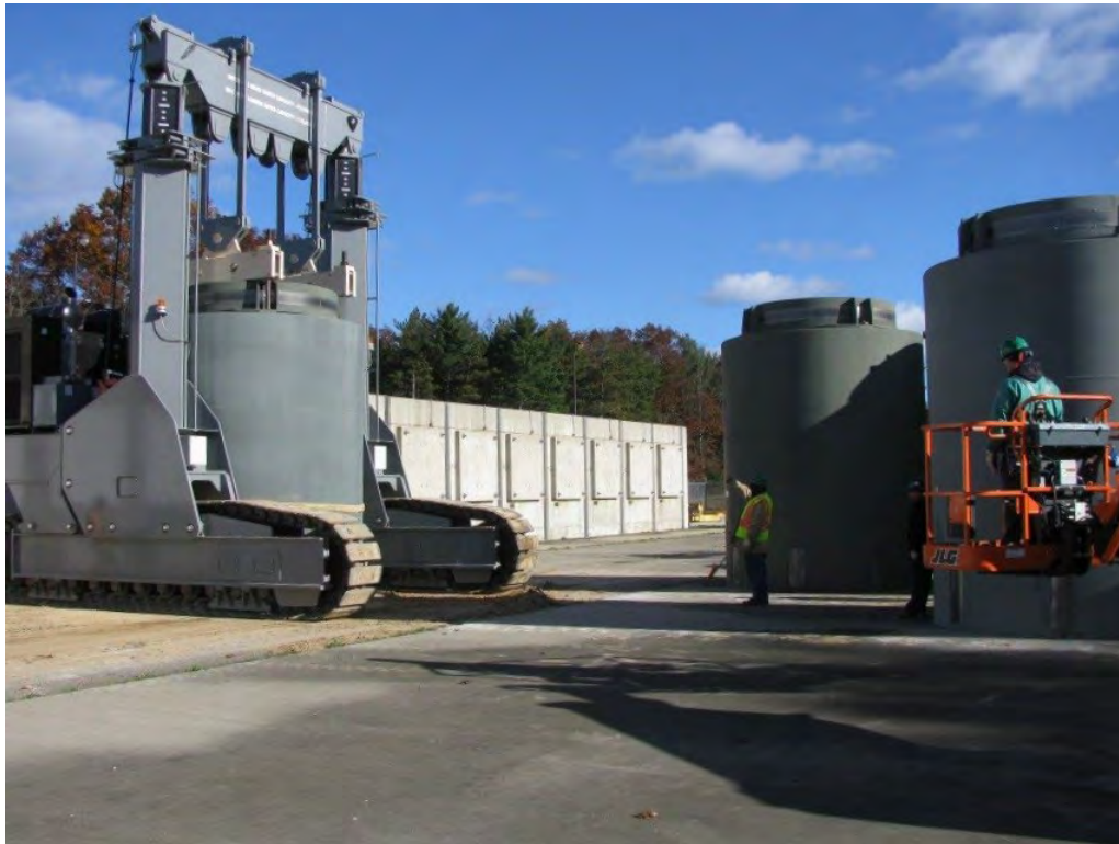
Figure 8. Canister and Vertical Concrete Overpack on ISFSI Pad
