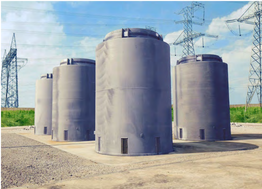
Figure 3. Vertical Canisters in Concrete Overpack
