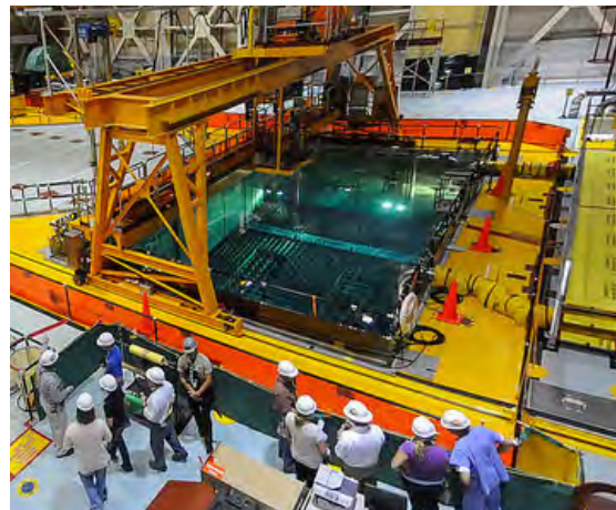
At least 23 feet of water covers the fuel assemblies in the spent fuel pool of Unit 2 at the Brunswick Nuclear Power Plant in Southport, NC. (Courtesy: Matt Born/Wilmington Star-News)
