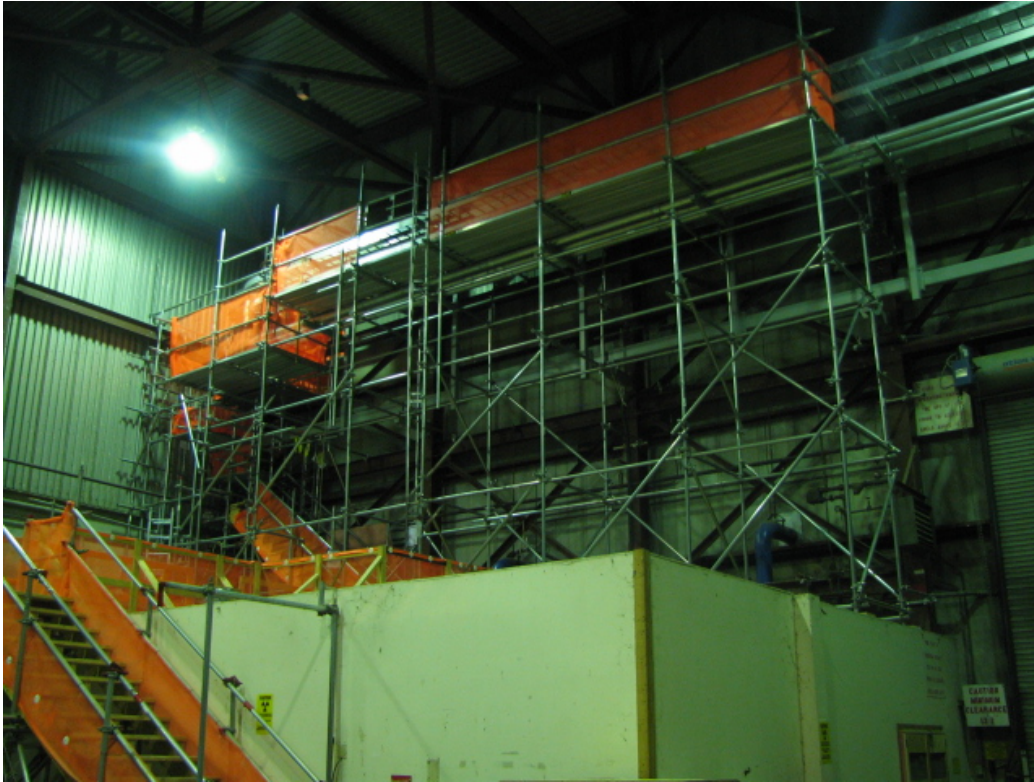
Scaffolding for 13.8 kV Raceway Installation in Turbine Building
