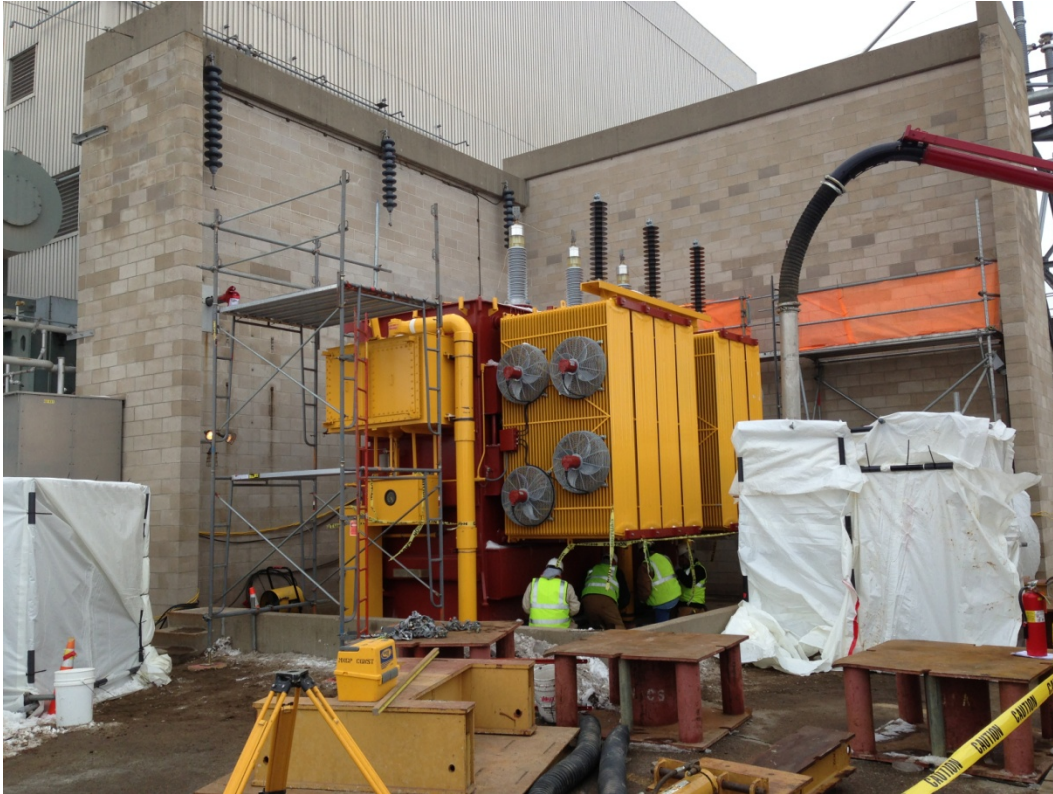
Installation of New 1R Transformer
