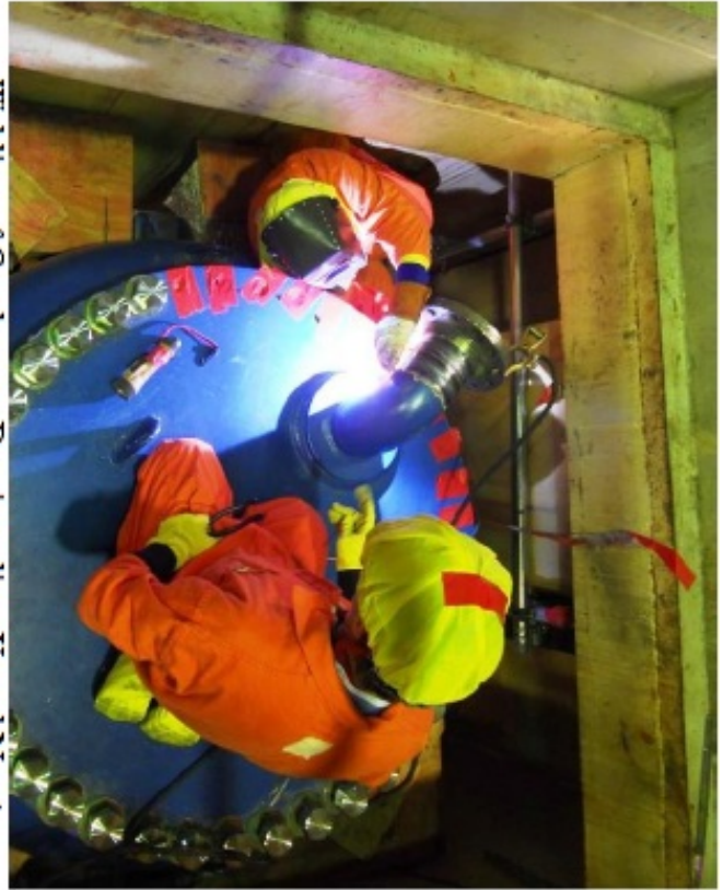
Welding of Condensate Demineralizer Vessel No. 4
