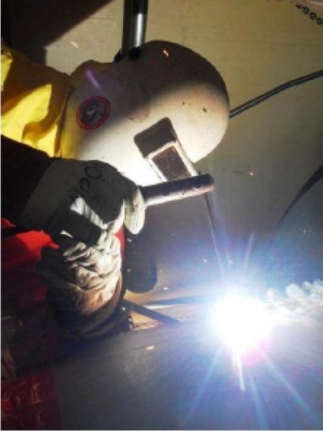
Welding Inside Condensate Demineralizer Vault
