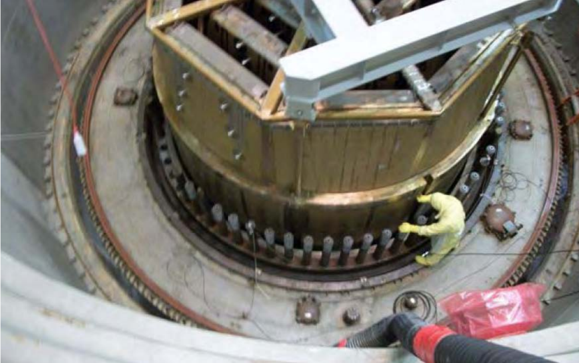
New Steam Dryer Being Set Into Reactor Vessel
