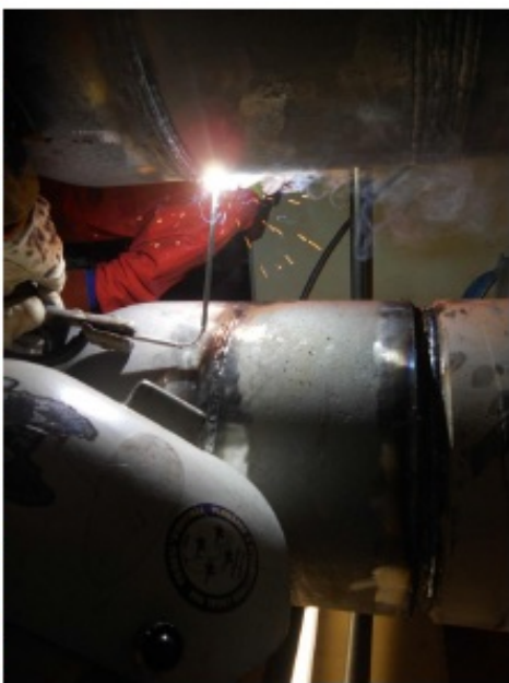
Welding Inside Condensate Demineralizer Vault
