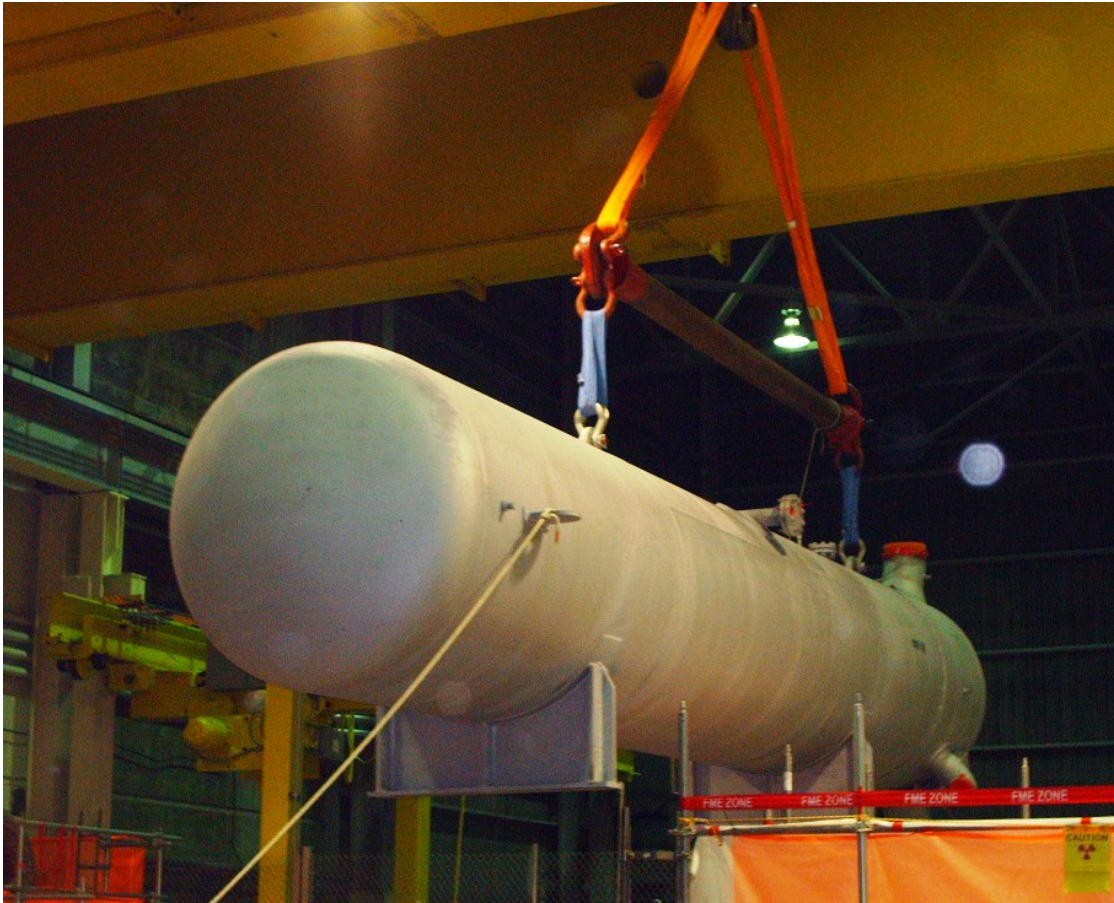
Arrival of Feedwater Heater 15A for Installation
