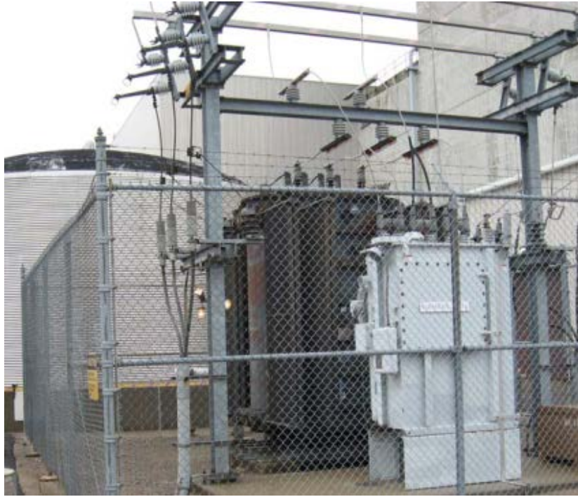
Existing 1AR Transformer Before Removal
