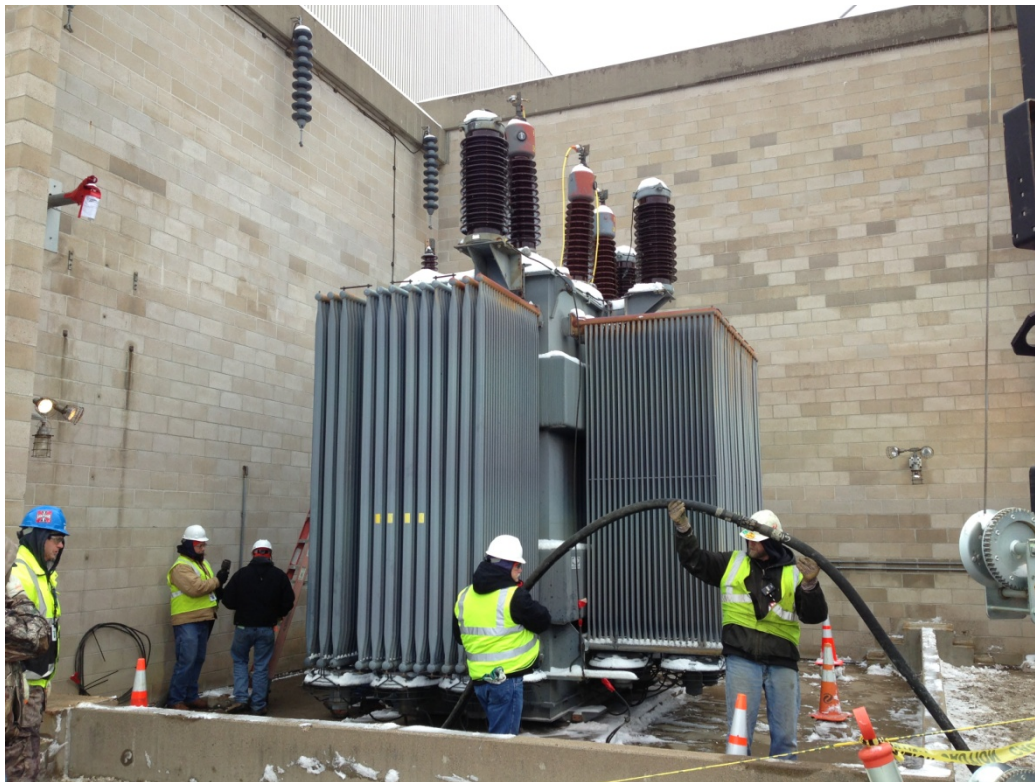
Existing 1R Transformer Removal
