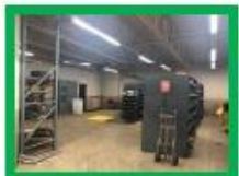
2. Material Storage - All Racking / Storage Shelves
