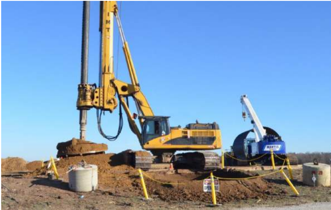
The diameter and depth of the hole depend on structure design and soil conditions Source: reference (7)
