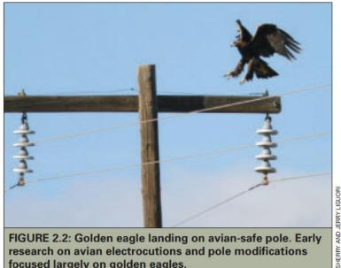
FIGURE 2.2: Golden eagle landing on avian-safe pole. Early research on avian electrocutions and pole modifications focused largely on golden eagles.
