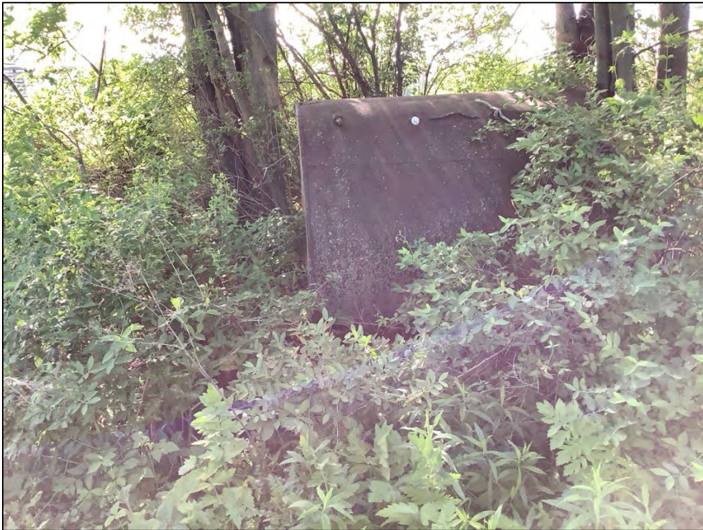
Photograph pp081 view of tank
