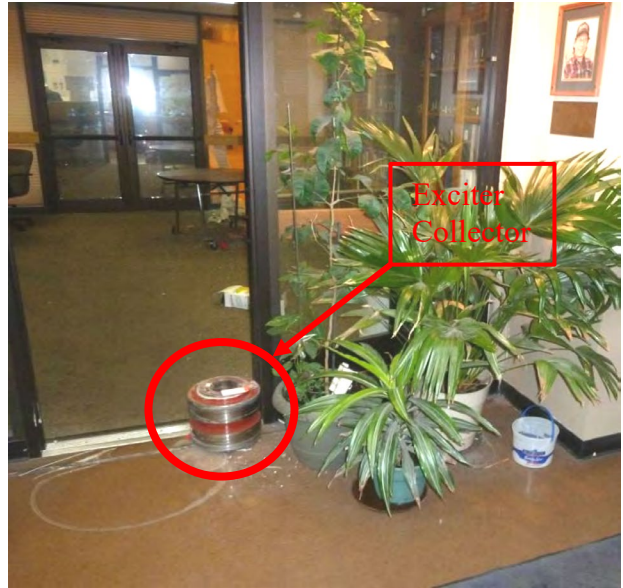
Figure 8 - Photograph of liberated exciter collector which came to rest in operator's room.
