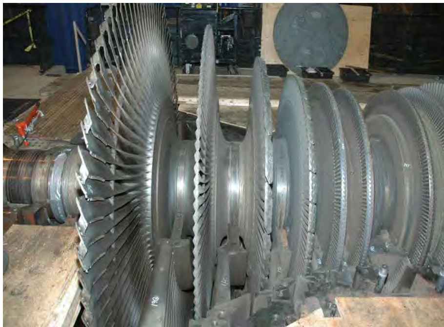
Fig. 69. Photograph of generator end of low pressure turbine "B" rotor.
