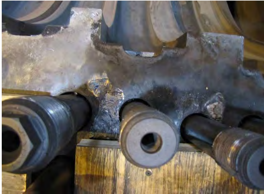
Fig. 28. Close-up of melting on intermediate pressure turbine inner casing shown in Fig. 27
