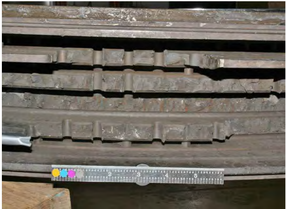
Fig. 123. Close-up photograph of fractures through internal finger pinned blade attachments of the low pressure turbine "B" L-1 disk rim.
