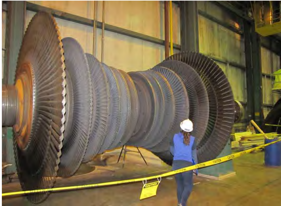
Fig. 44. Photograph of low pressure turbine rotor "A" in stands at site.
