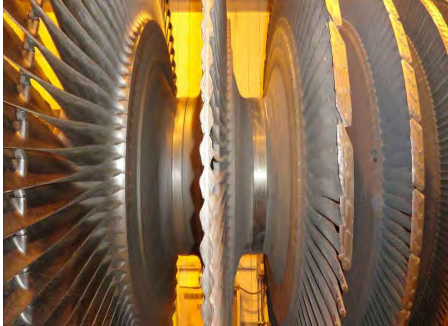
Fig. 70. Photograph of generator end of low pressure turbine "B" showing damage to shrouds on L-1, L-2 and L-3 stages.
