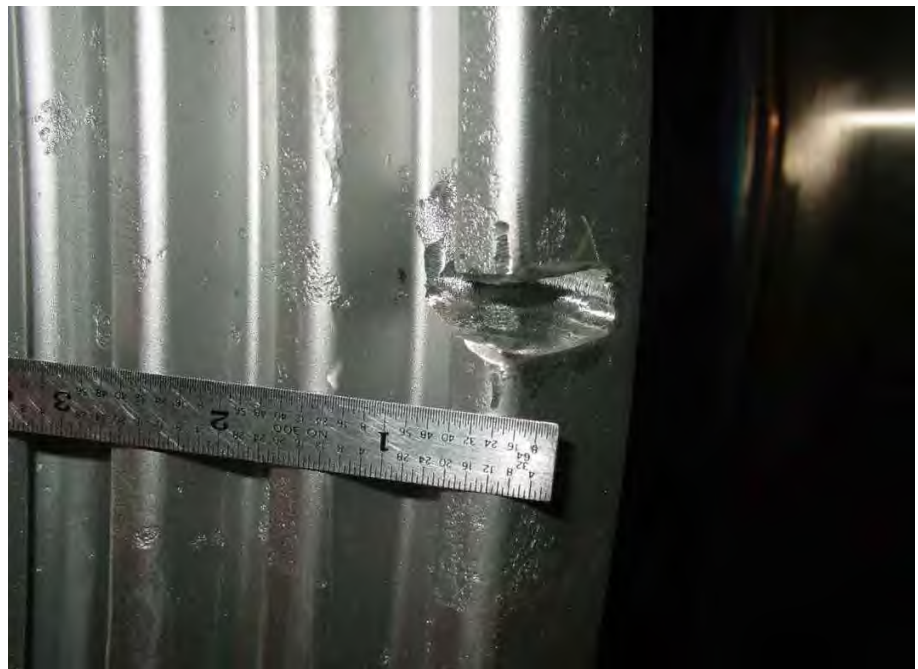
Fig. 103. Close-up photograph of low pressure turbine "A" generator end L-2 stage disk rim showing excavation of indication at 155° location.
