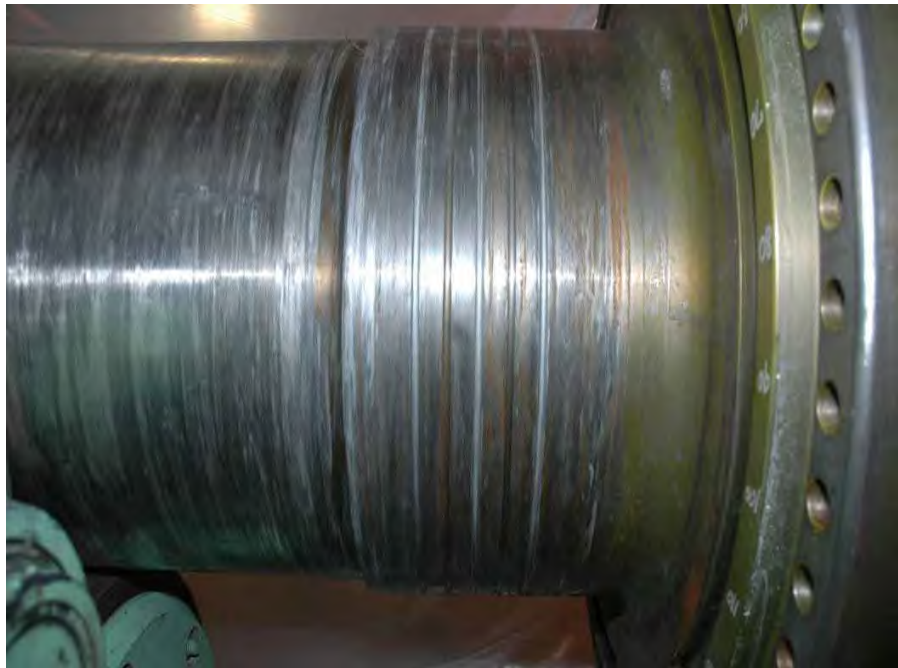
Fig. 113. Generator rotor rub damage.
