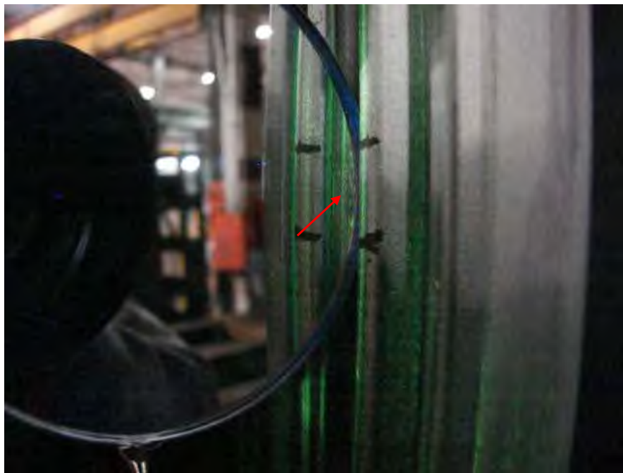
Fig. 95. Close-up blacklight photograph of low pressure turbine "A" generator end L-4 stage disk on the inlet side of the blade dovetail showing indication (arrow).
