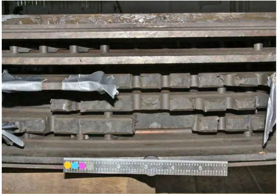
Fig. 122. Close-up photograph of fractures through internal finger pinned blade attachments of the low pressure turbine "B" L-1 disk rim.
