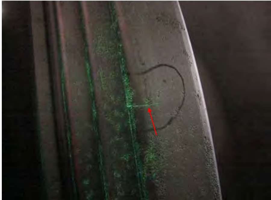
Fig. 92. Close-up blacklight photograph of low pressure turbine "A" generator end L-2 stage disk on inlet side of the blade dovetail showing indication (arrow).
