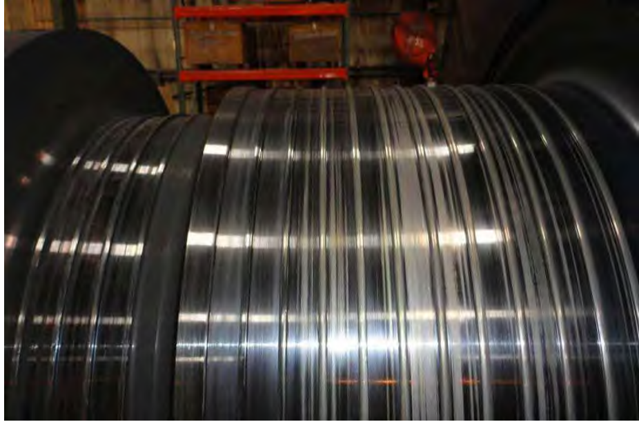
Fig. 36. Close-up photograph of intermediate pressure turbine showing rub damage on seal surface.
