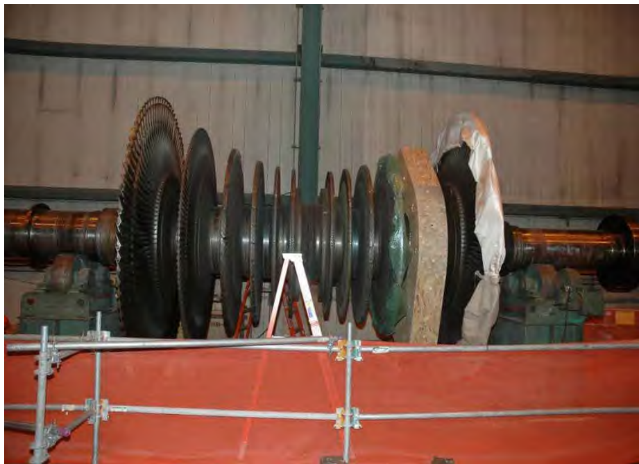
Fig. 83. Photograph of low pressure turbine "B" rotor with wooden protective box built around the fractured L-1 stage disk rim.
