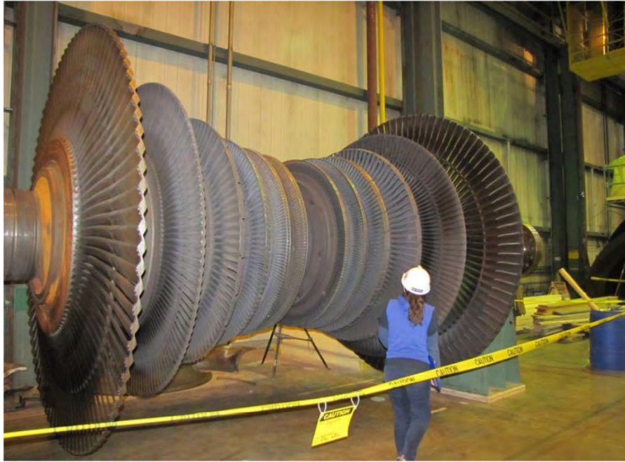
3 Figure 1 4 Photograph of Unit 3 low pressure turbine rotor “A” 5 in stands at the Event site
