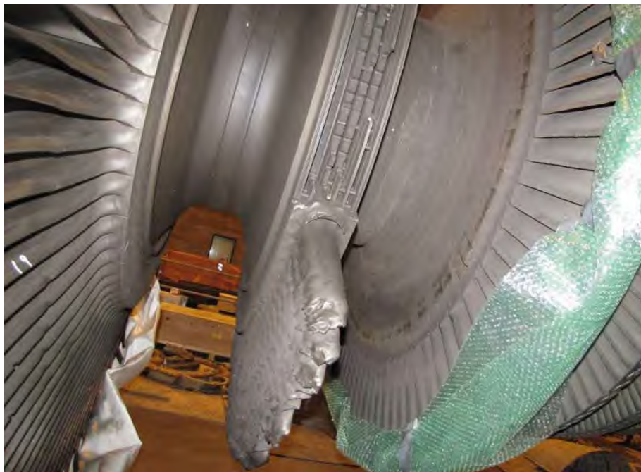
Fig. 59. Close-up of fractured turbine end L-1 stage disk section of low pressure turbine "B" rotor shown in Fig. 55.
