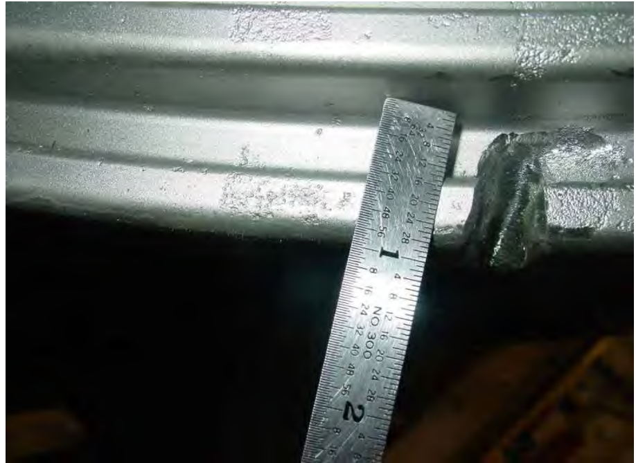
Fig. 100. Close-up photograph of low pressure turbine "A" generator end L-2 stage disk rim showing excavation of indication at 330° location. Viewed from side.
