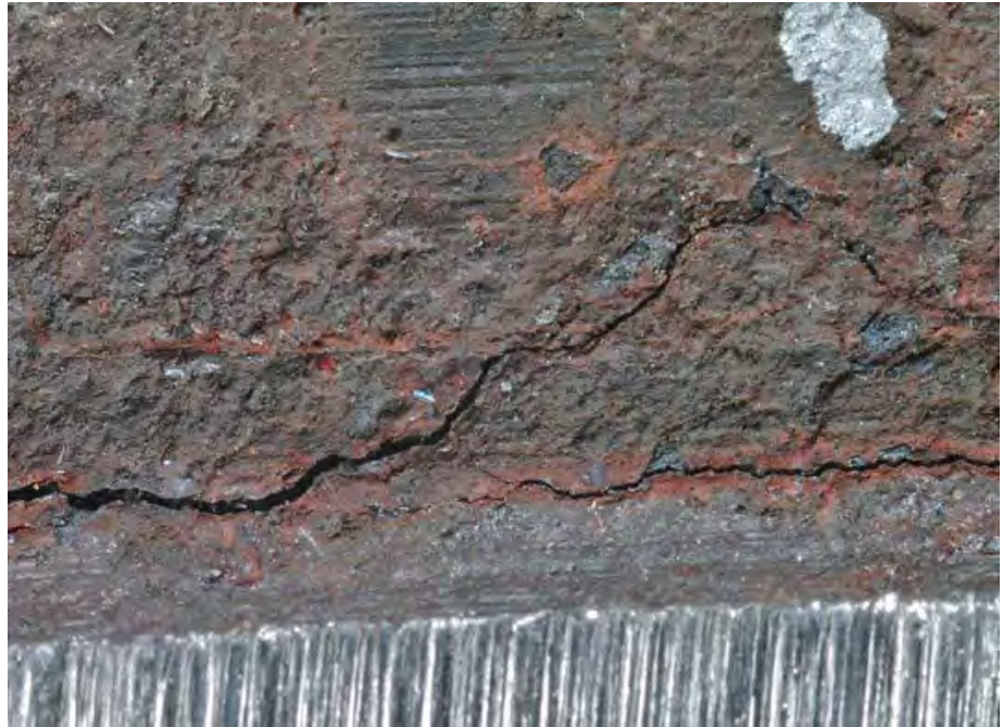
Fig 160. Close-up of SID 14875 subsegment "C4" crack No. 1 shown in Fig. 158, viewed from inlet side.
