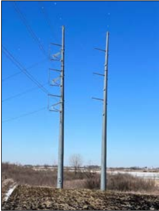
Figure 2.5-4 Typical Configuration of Two Monopole Structures Side-by-side
