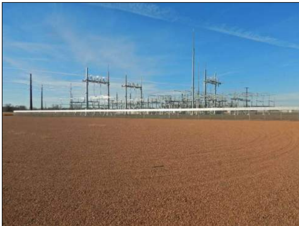
Figure 94: View facing southwest towards site 21RN0038 (DSCN8814).
