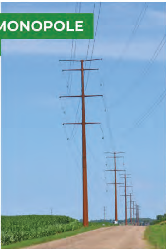
Image shown is an example of a similar double-circuit structure.
