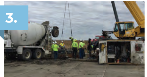
Foundation Drilling & Pouring
