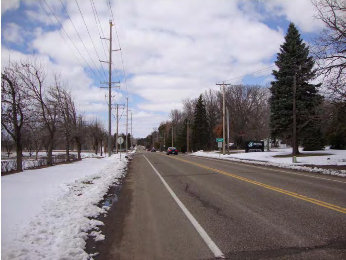
Figure 11. Existing Distribution Line Underbuild along Otter Lake Road 129
