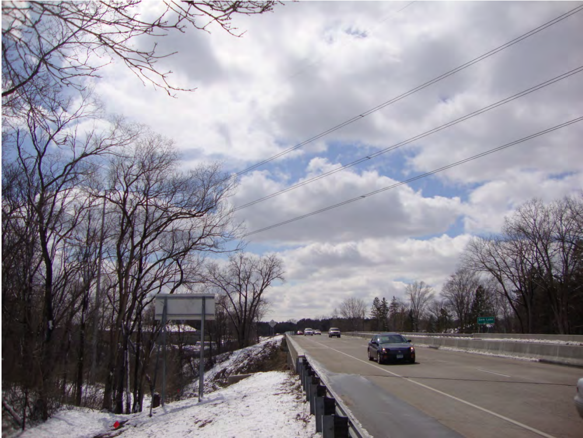
Figure 10. Existing Single Circuit 115 kV Crossing of Highway 61
