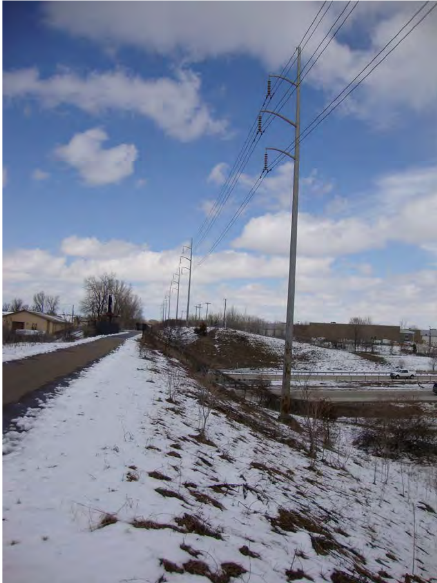
Figure 9. Existing Single Circuit 115 kV Crossing of I-694 123
