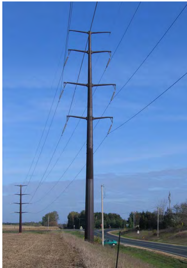
Figure 6. Double Circuit Davit Arm Structure 35
