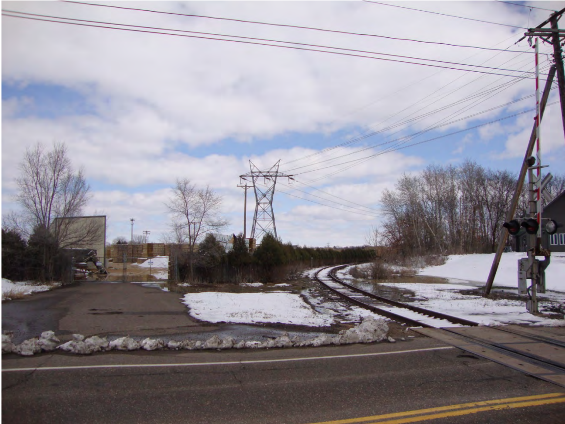
Figure 8. Existing Single Circuit 115 kV Lattice Tower Structure 43
