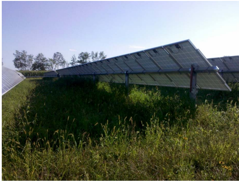
Figure 1: Typical solar tracker row design.
