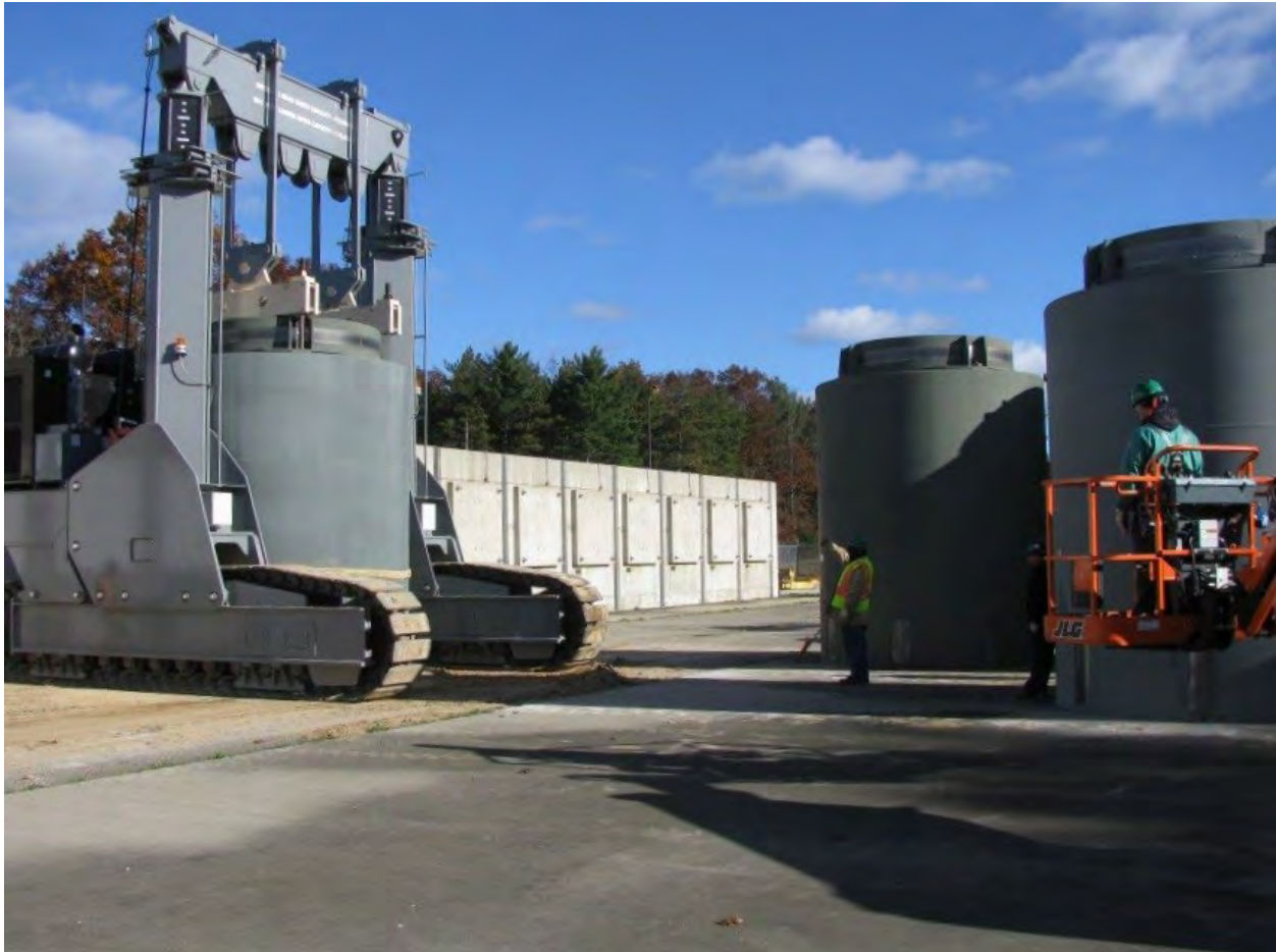
Figure C-14: Overpack and Canister Movement to ISFSI Pad Using Transporter
