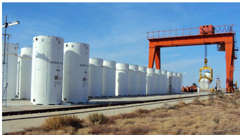
At right, a dry storage cask recently loaded with spent fuel is lifted from a horizontal transporter to be placed on a specially designed storage pad. (Courtesy: Sandia National Laboratories)
