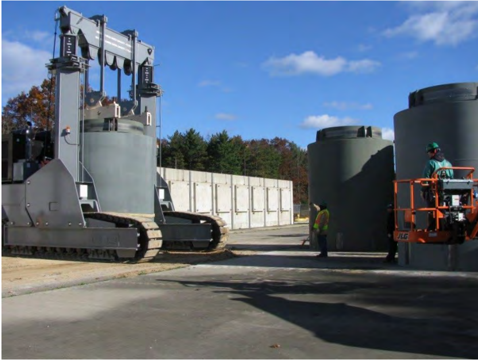
Figure 7. Canister and Vertical Concrete Overpack on ISFSI Pad
