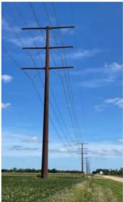
Figure 3-2 Representative Monopole Structure
