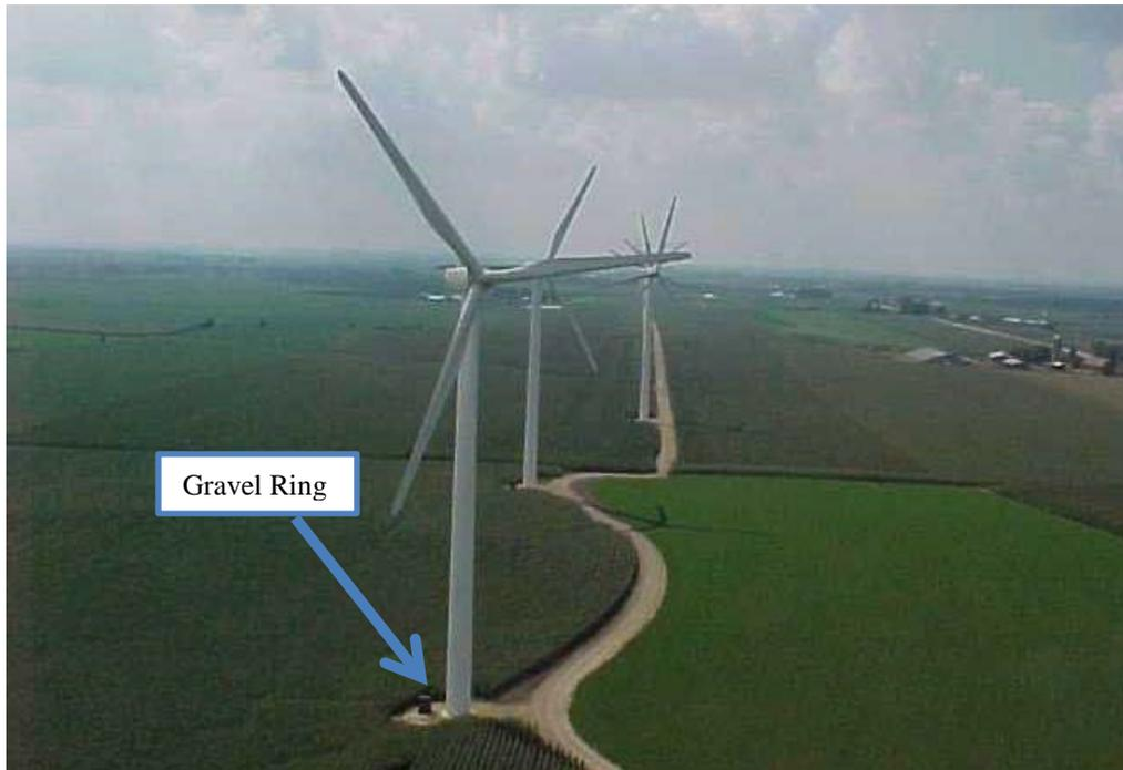
The typical cross section of access roads will be dependent on terrain, grade, and drainage considerations. Access roads may incorporate geotechnical fabric and cement stabilization measures beneath the aggregate roadway cap. Also, if necessary, a final aggregate dressing may be placed on some of the turbine access roads.
