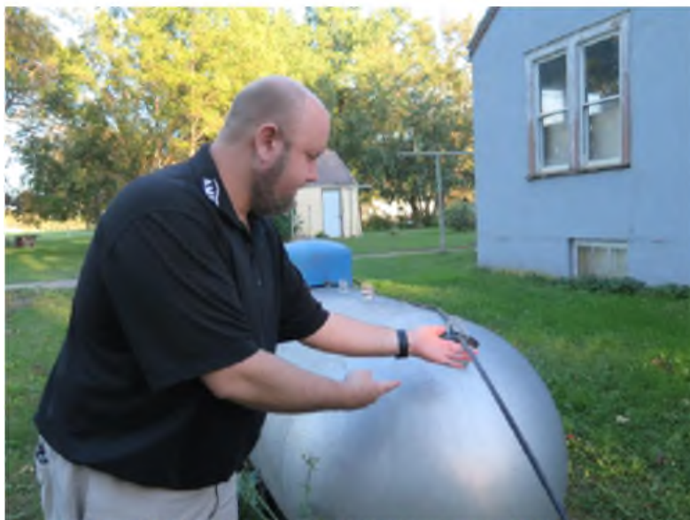
Ceylon City Council Member John Gibeau says Frontier Communications failed to complete this telephone line project. The cables have not been buried or attached to poles. This one crosses a propane gas tank. Mark Steil | MPR News
