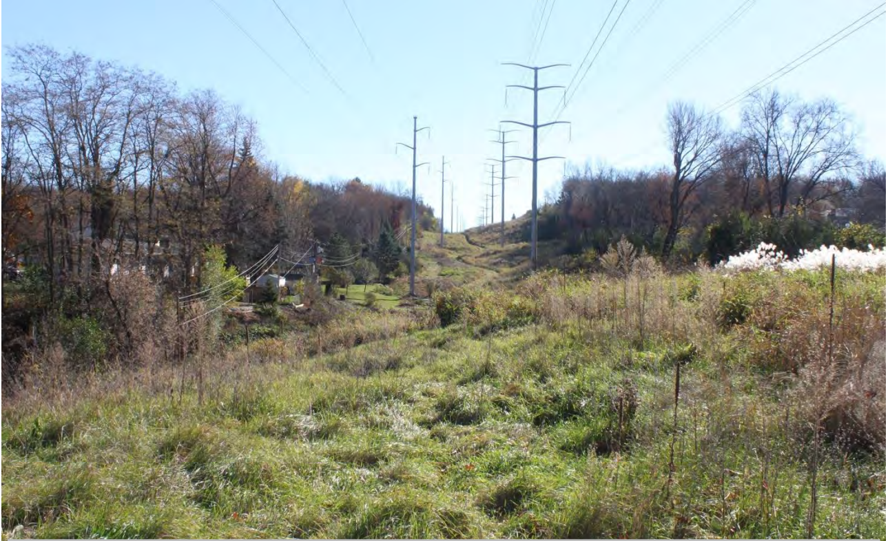
View back to the SE from bluff above railroad tracks, maintenance road visible in the distance between transmission line poles
