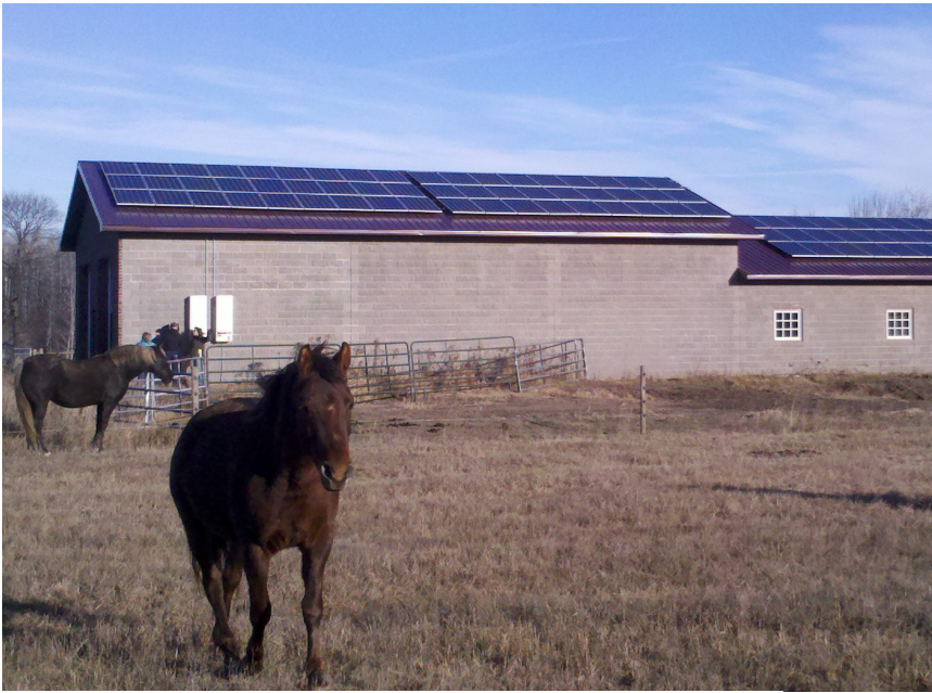
Photo: Pine City, MN (21 kW, 2012) Photographer: Dan Williams
