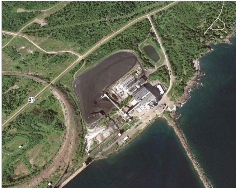
Figure 3.4: THEC Site Aerial
