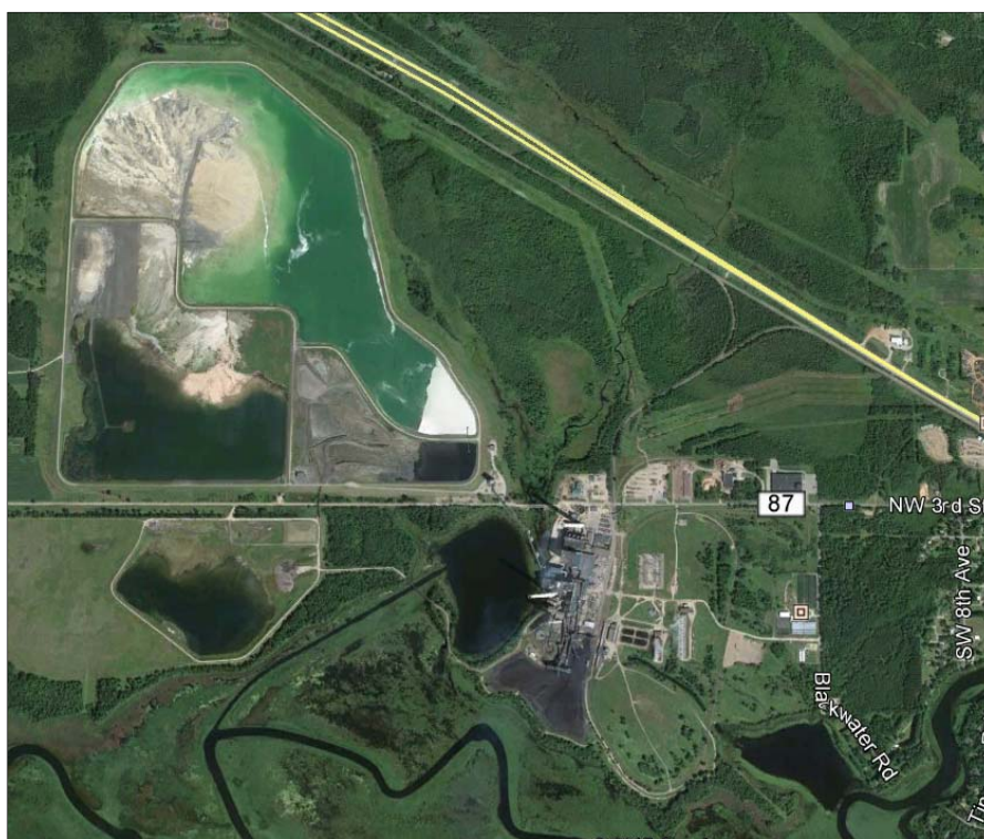
Figure 3.1: BEC Site Aerial
