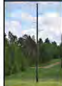
Typical 115 kV Wood Single Circuit Structure
