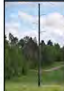
Typical 115 kV Wood Single Circuit Structure
