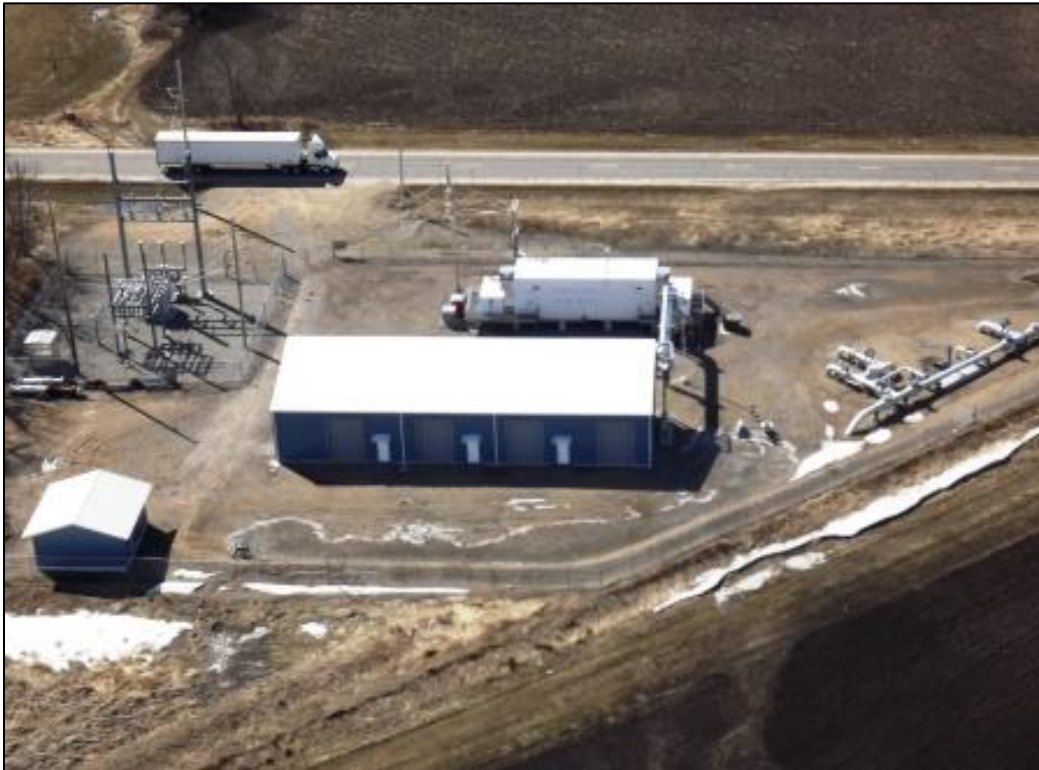
Figure 1. Existing Pumping Station near Albany, Minnesota 9
