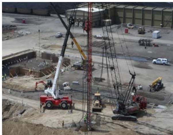
05-07 Production piles south SCR tower
