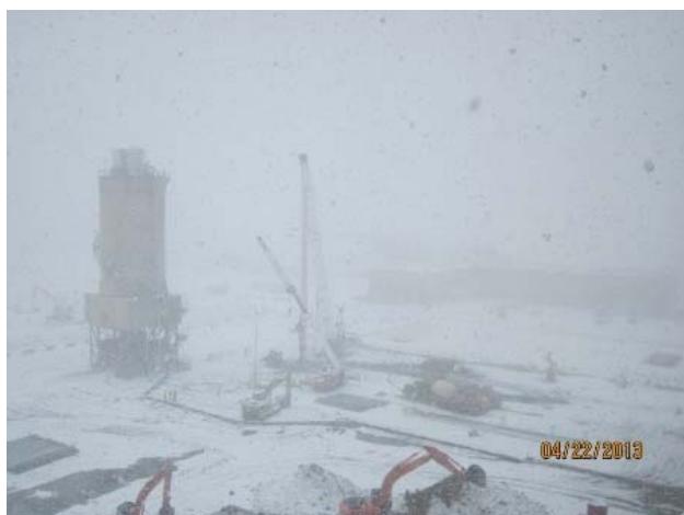
04-22 Waste ash/pebble lime silo
