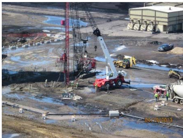
04-19 Auger cast pile installation waste ash/pebble lime silo
