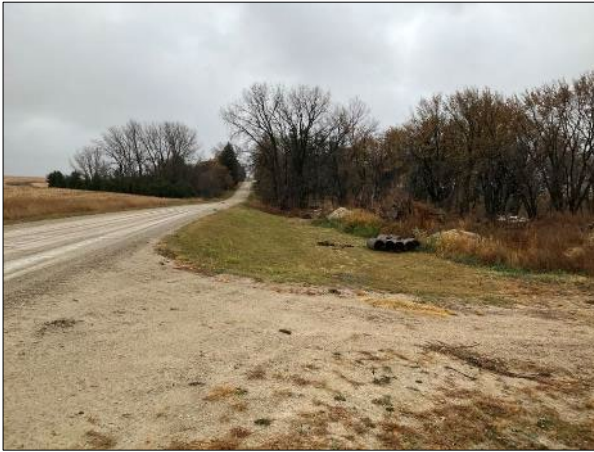
Photo 5.4-5. Overview of road and ROW, facing south.
