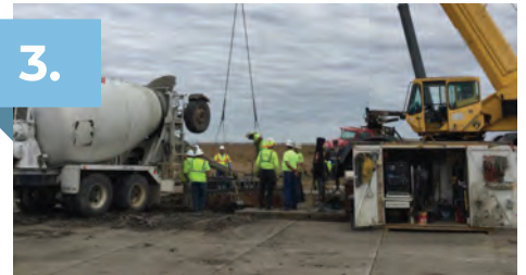
Foundation Drilling & Pouring
