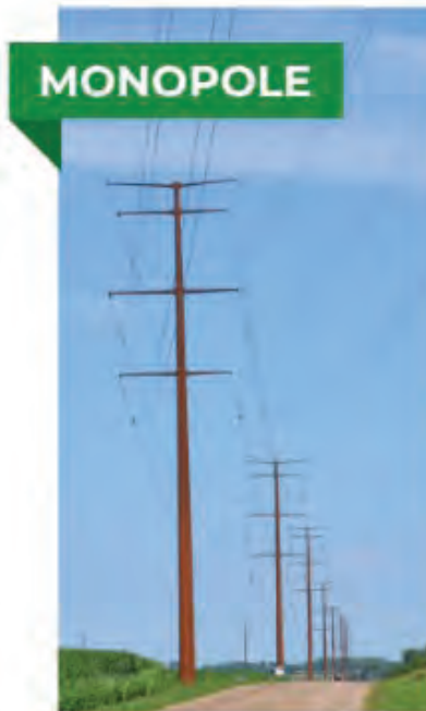
Image shown is an example of a similar double-circuit structure.
