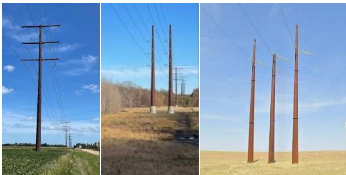
Typical Double-Circuit Structures
