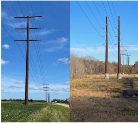
Typical Double Circuit Structures | Typical Dead-end Structures
