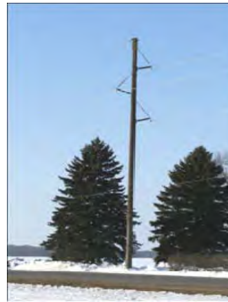
Typical Braced Post 115 kV Structure
