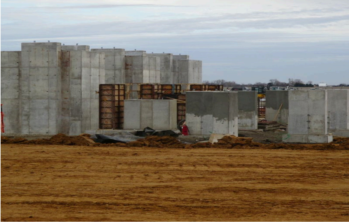
Decatur - Electrical Service Building (ESB) Foundation Formed Up
