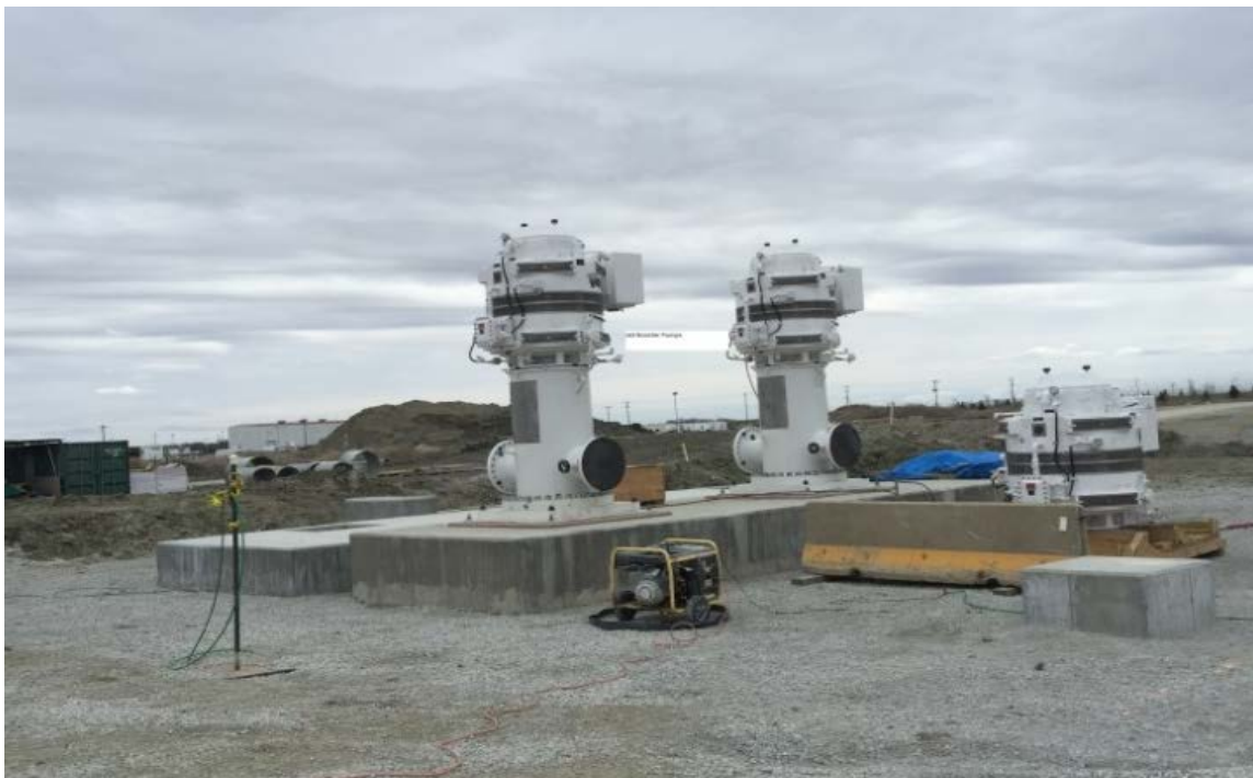
Flanagan Terminal / Pump Station - Terminal Side Booster Pump Installation
