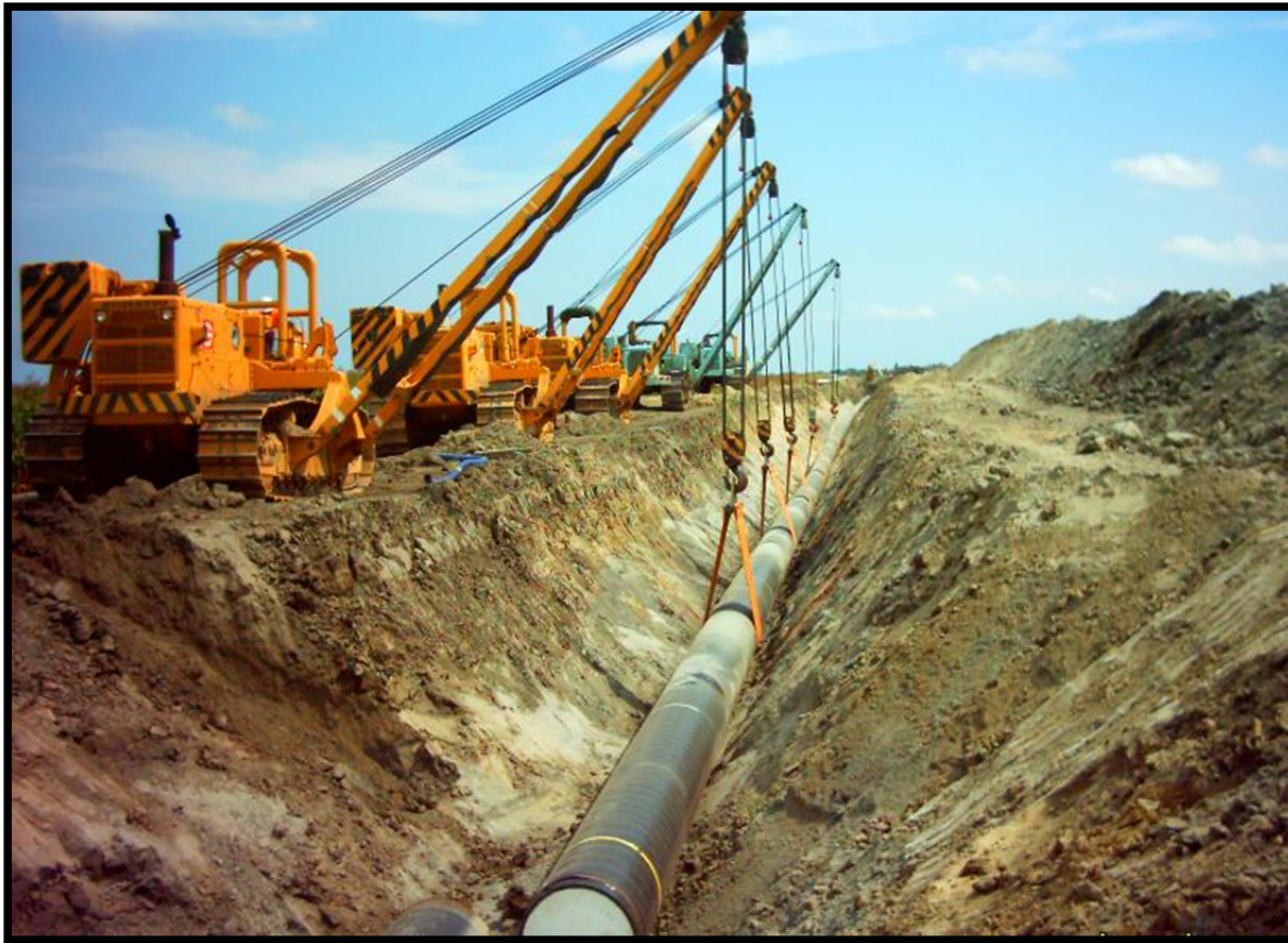
Figure 4.2.6-1 Lowering of the Pipeline
