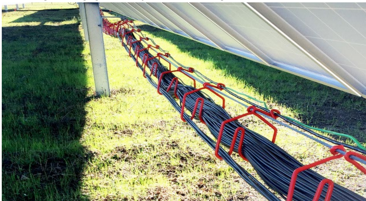
Image 2: Hanging Harness System for DC Cabling between Panels and Inverters
