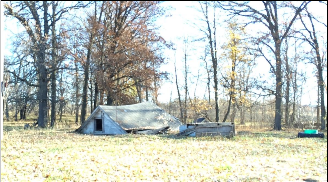
Figure 28. Structural remains at site 21CE0079, facing southeast.
