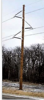
Diagram 3-2. Photos of Typical 115-kV Transmission Structures
