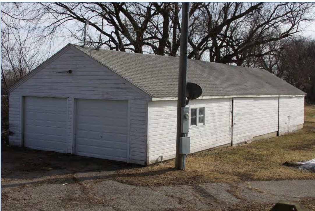
Figure 49. Northwest corner angle of Feature 2. View to the southeast.
