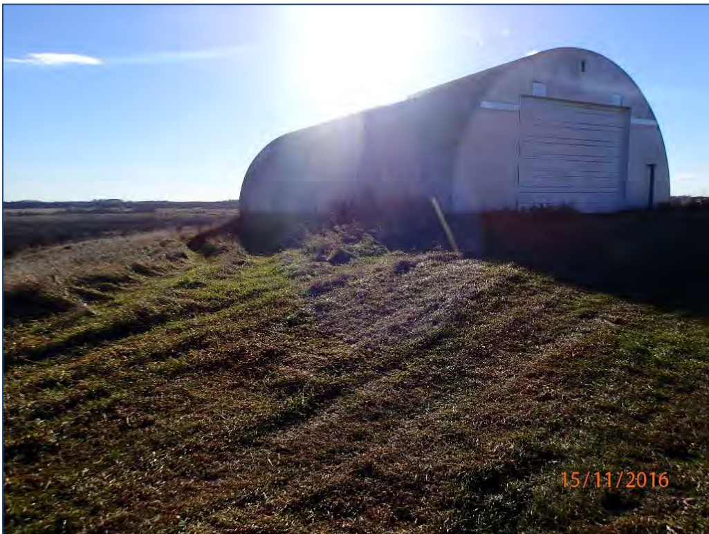
Figure 40. Feature 7: Metal shed view to the southwest.
