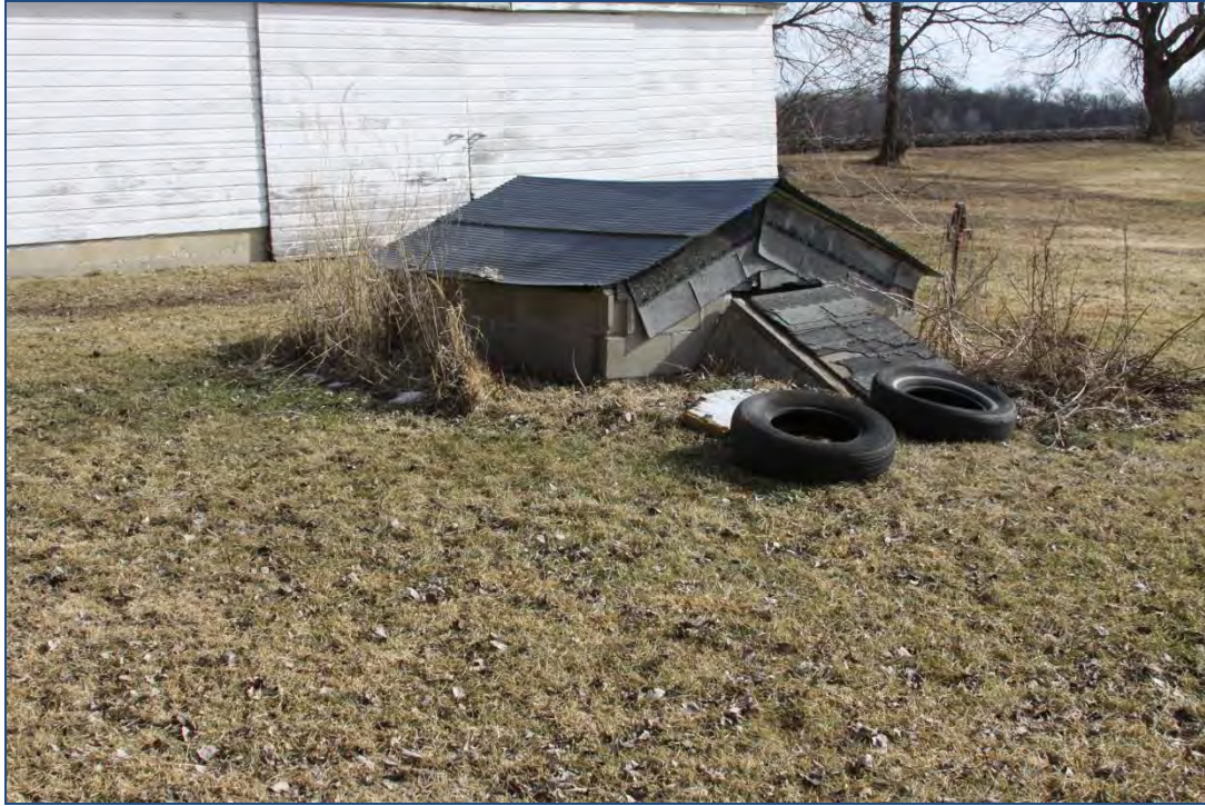
Figure 50. Northwest corner angle of Feature 3. View to the southeast.
