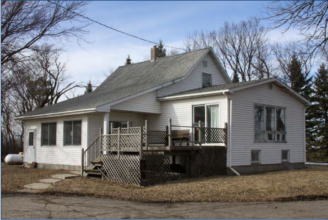
Figure 48. Southeast corner angle of Feature 1. View to the northwest.
