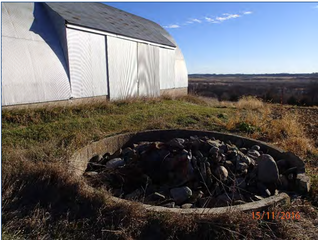
Figure 36. Feature 4 and Feature 7: Silo foundation and metal shed view to the southeast.
