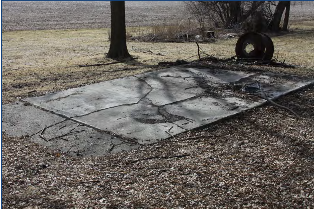
Figure 56. A modern concrete pad. View to the southwest.
