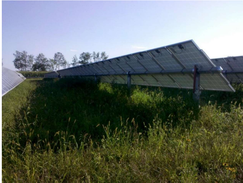
Figure 3 : Typical Solar Tracker Row Design
