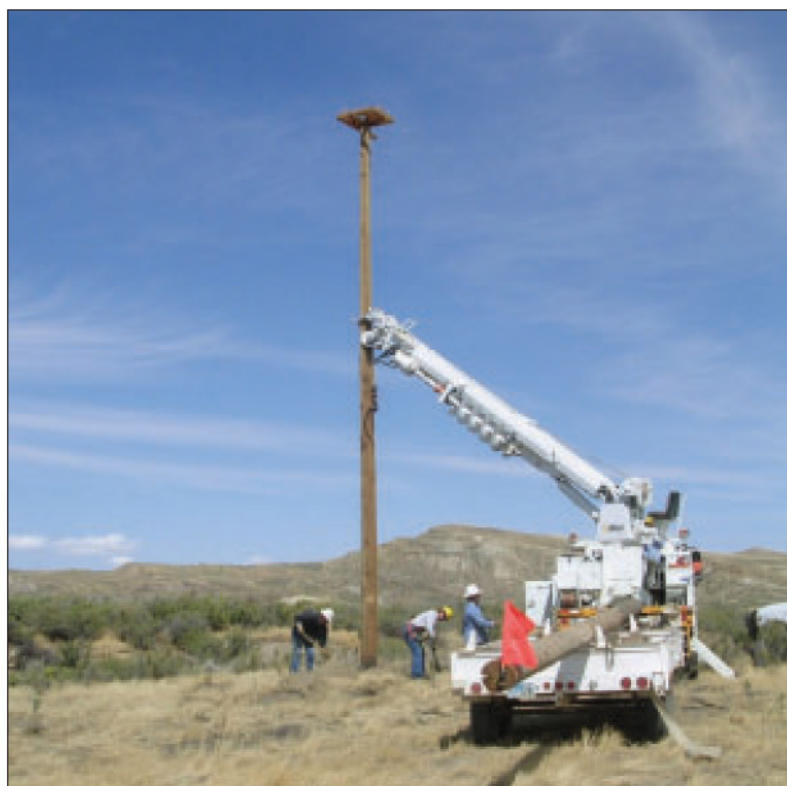
FIGURE 7.1: Utility crew installing raptor nest platform.
