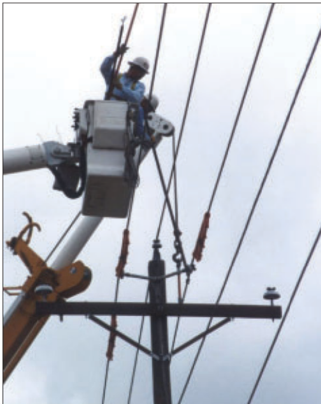
FIGURE 7.2: Reframing a crossarm to prevent avian electrocutions.
