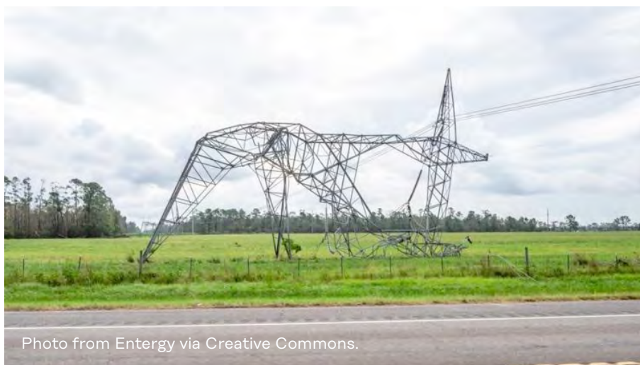
Figure 9. Damage from Hurricane Laura on overhead transmission
