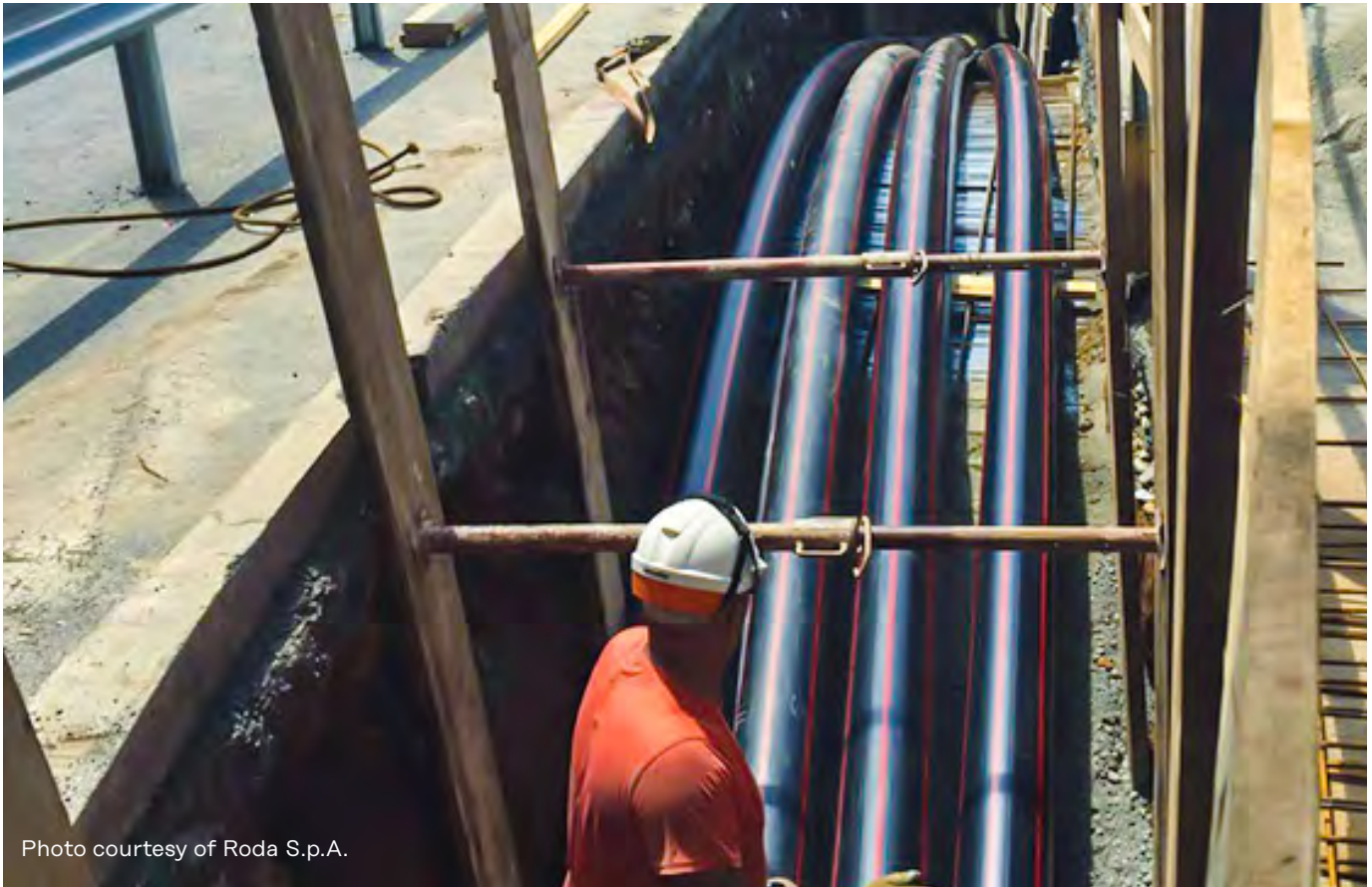
Figure 2. Buried HVDC cables in highway ROW (Italy-France Interconnector)
